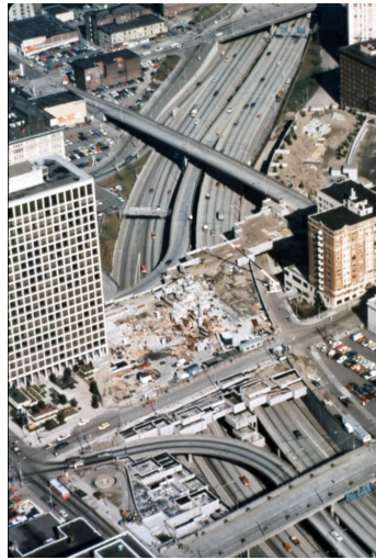
Aerial showing Freeway Park under construction, circa 1975. Image 203829 , Series 1629-01, SMA.
