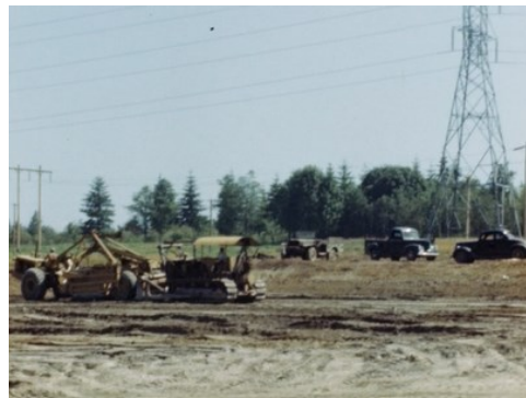
B-roll of workers excavating land for construction of the Bothell Substation, August 1948. Event 142 , Series 1204-05, SMA.
