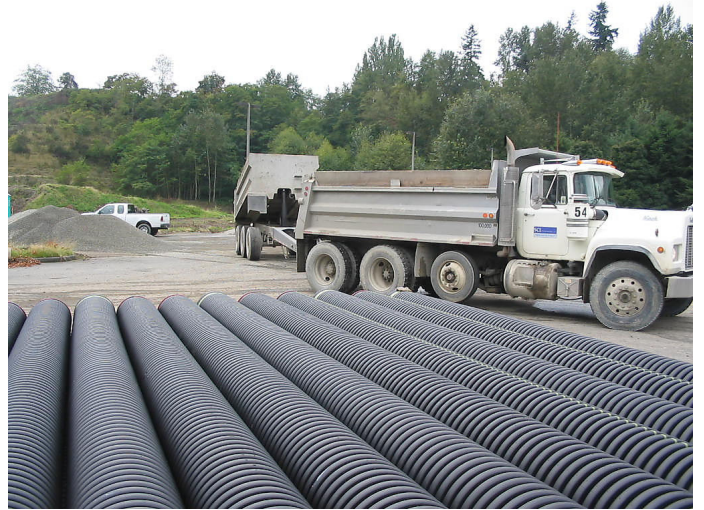
Early site construction, September 2004. Item 159357, FFD Capital Programs Division Photos, Seattle Municipal Archives
