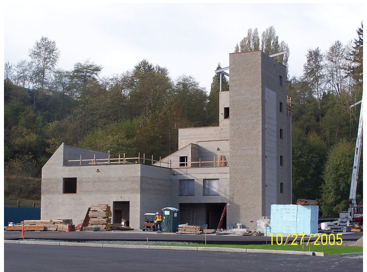
Drill Tower Construction, October, 2005. Item 159357, FFD Capital Programs Division Photos, Seattle Municipal Archives
