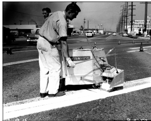
New paint machine in use at First Ave S. and E. Marginal Way, September 11, 1957
