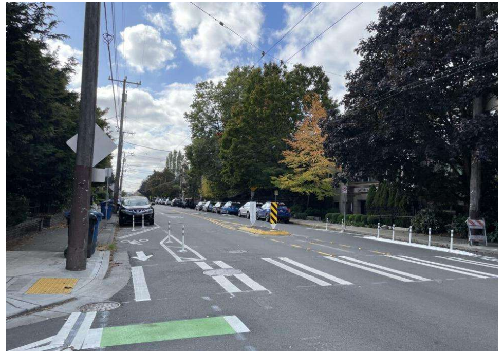
New speed cushions and signed crosswalk at 10 th Ave E and E Highland Drive.
