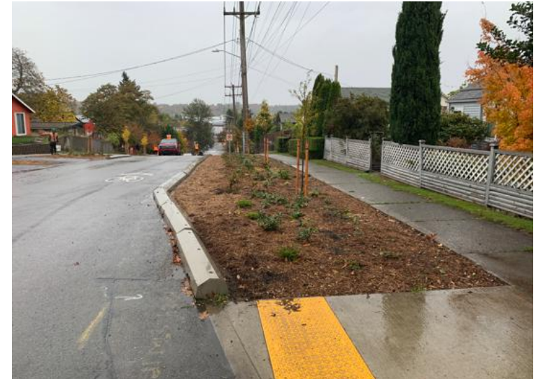
Wheel Stops and Conveyance Swales
