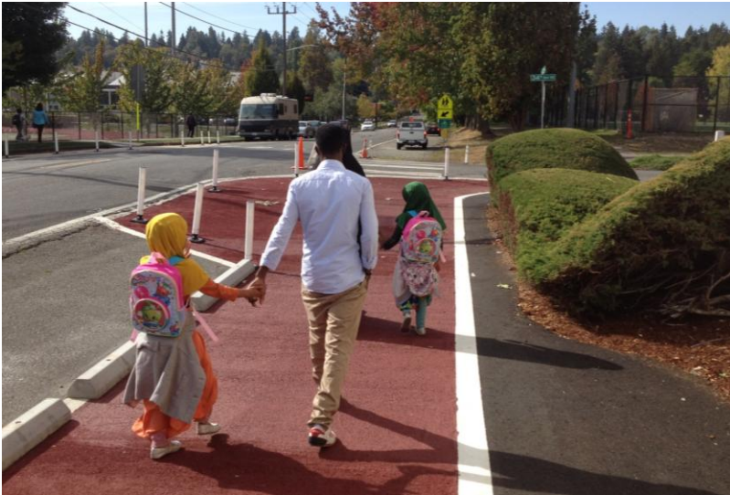
Painted Walkways with Wheel Stops
