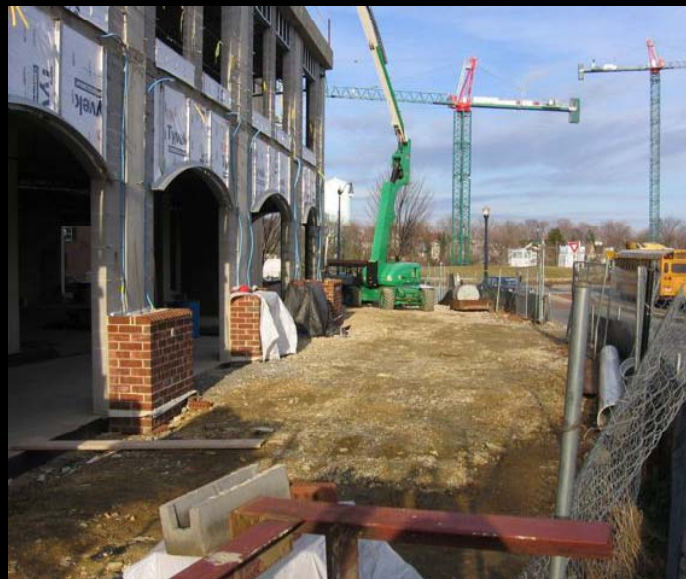
Construction on disturbed soils
