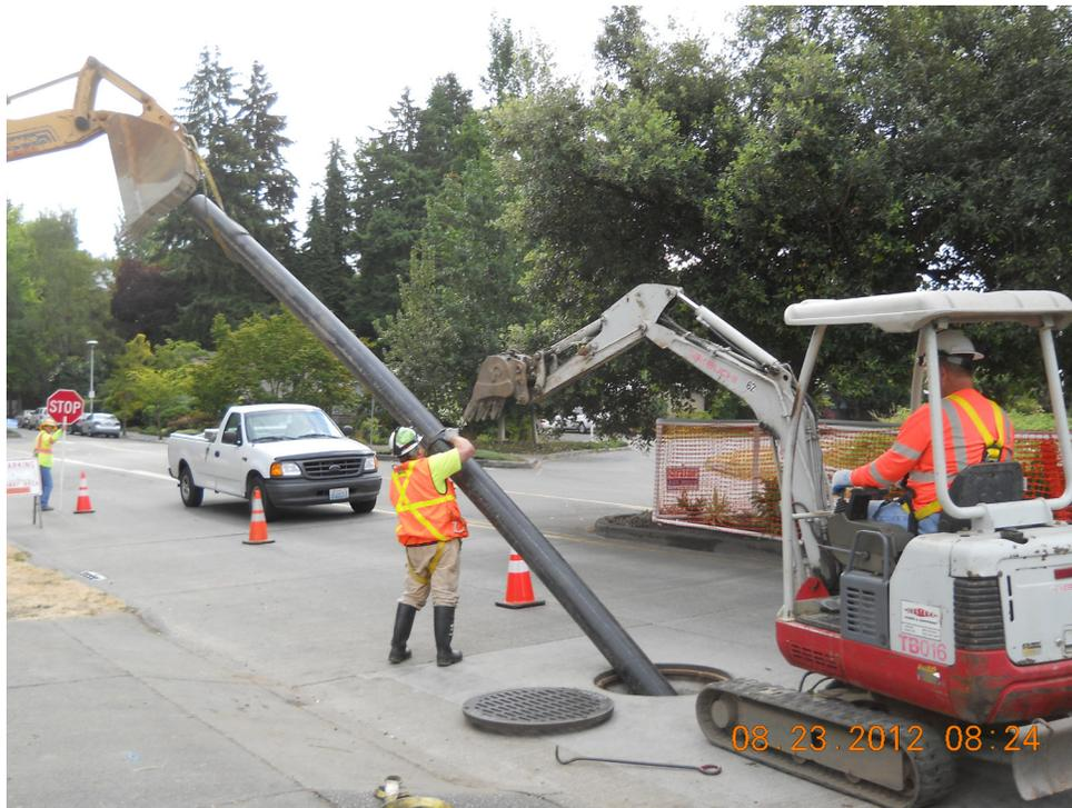
Figure 4-3. New Side Sewer Interceptor Pipe (North Union Bay Area)
