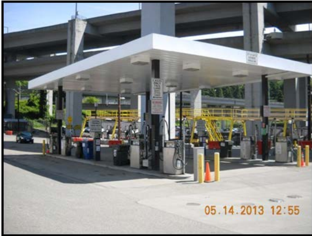
Figure 8. Roof at Fueling Island to Prevent Stormwater Run-on.
