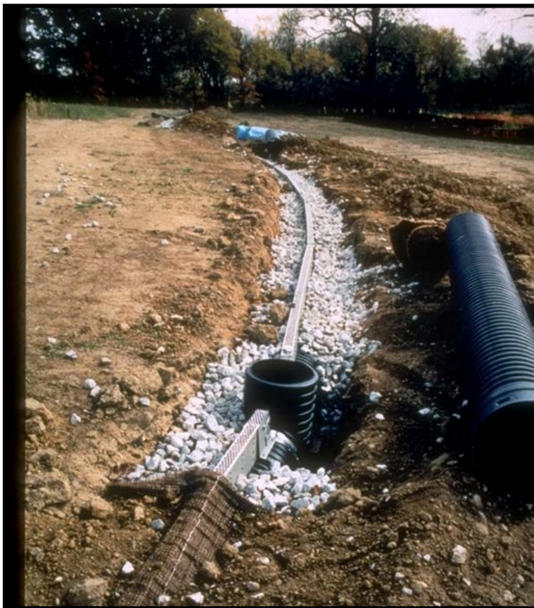
Figure E.6. Level Spreader Prior to Backfill and Downstream Stabilization.
