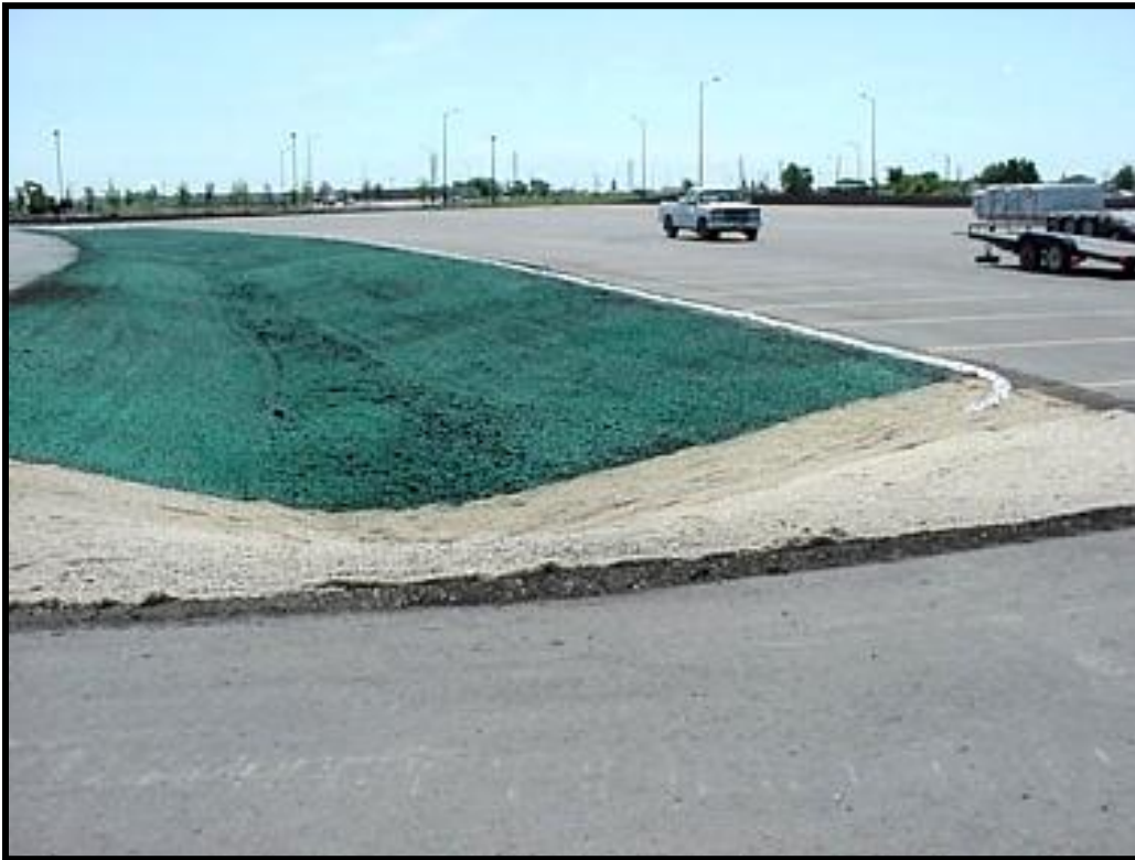
Figure 1. Hydroseeding Method.
