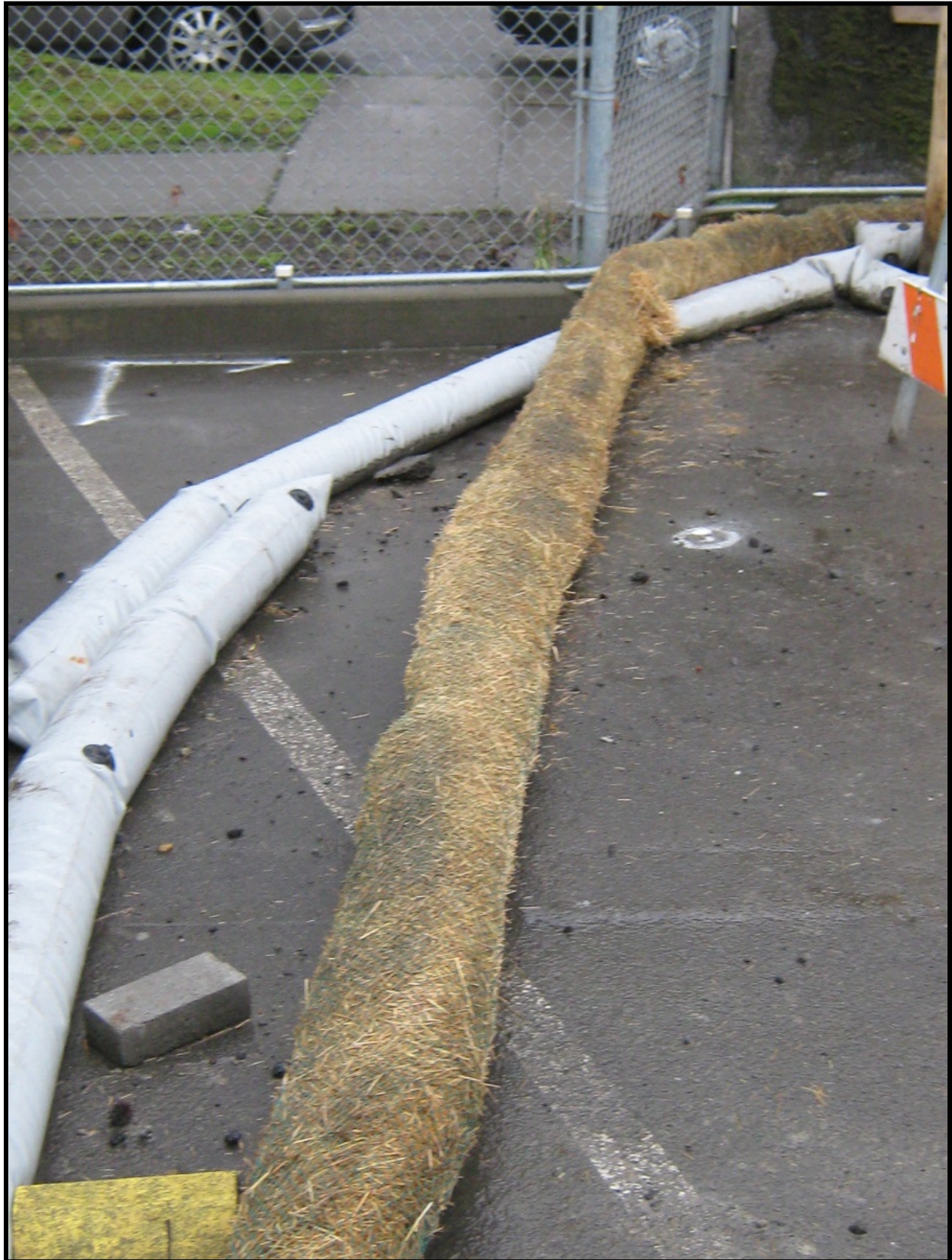
Figure 16. Curb and Gutter Barrier.
