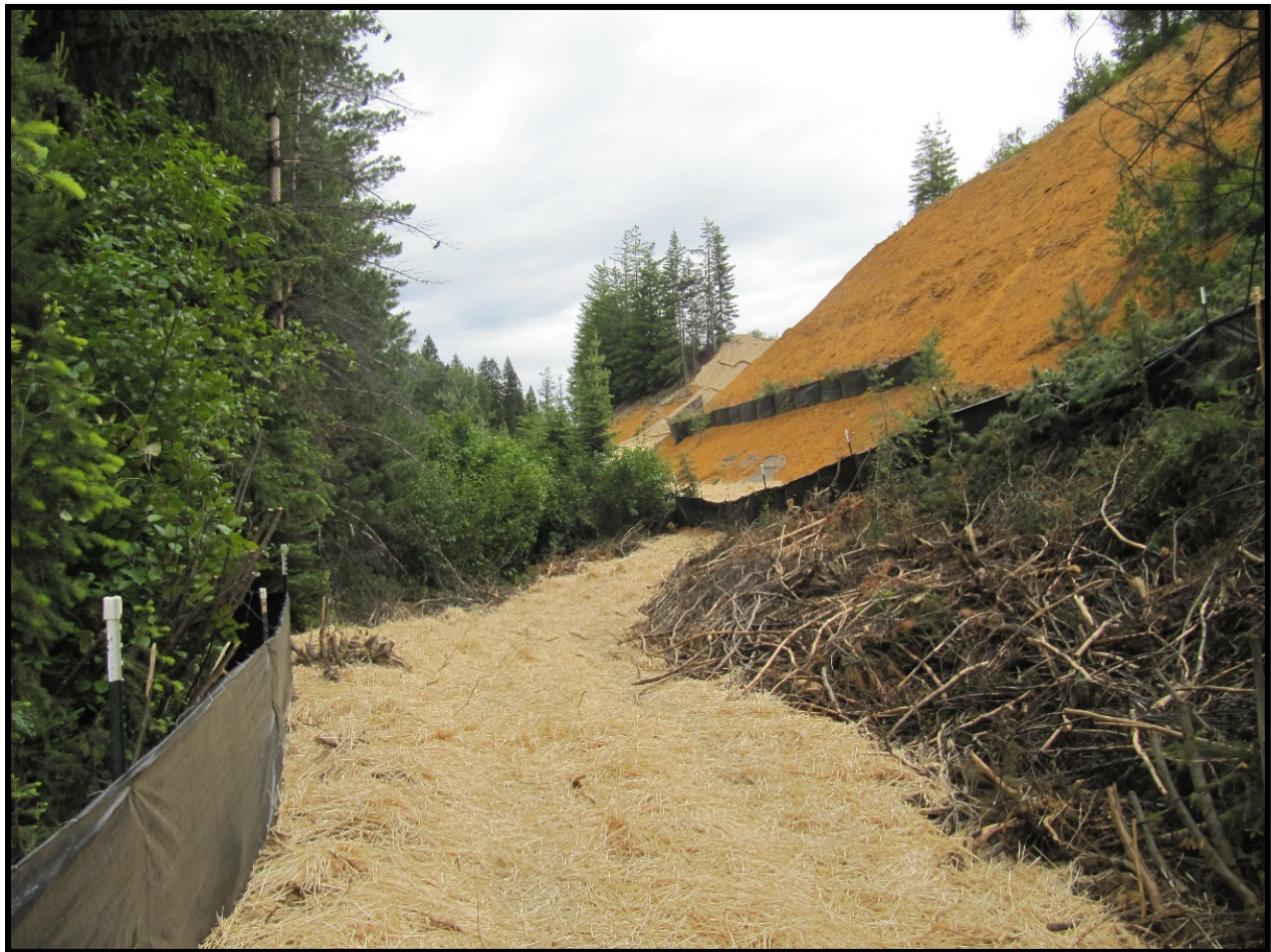
Figure 13. Filter Fence Installed on a Slope.
