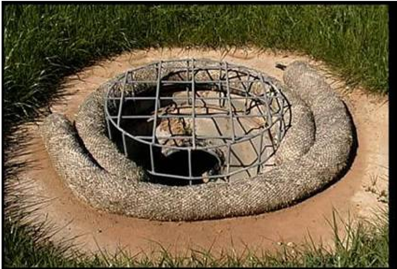
Figure 17. Straw Wattles or Compost Sock for Inlet Protection.
