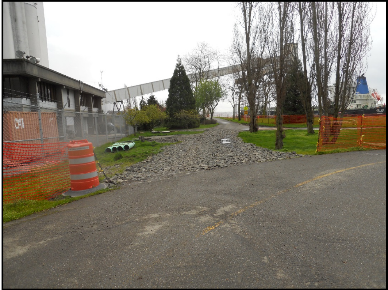
Figure 7. Stabilized Construction Entrance.
