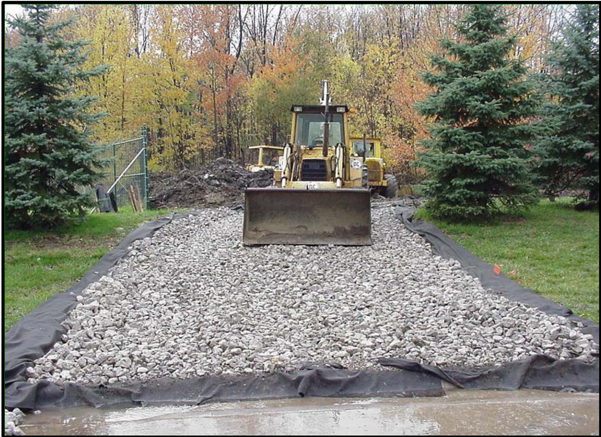
Figure 6. Stabilized Construction Entrance.
