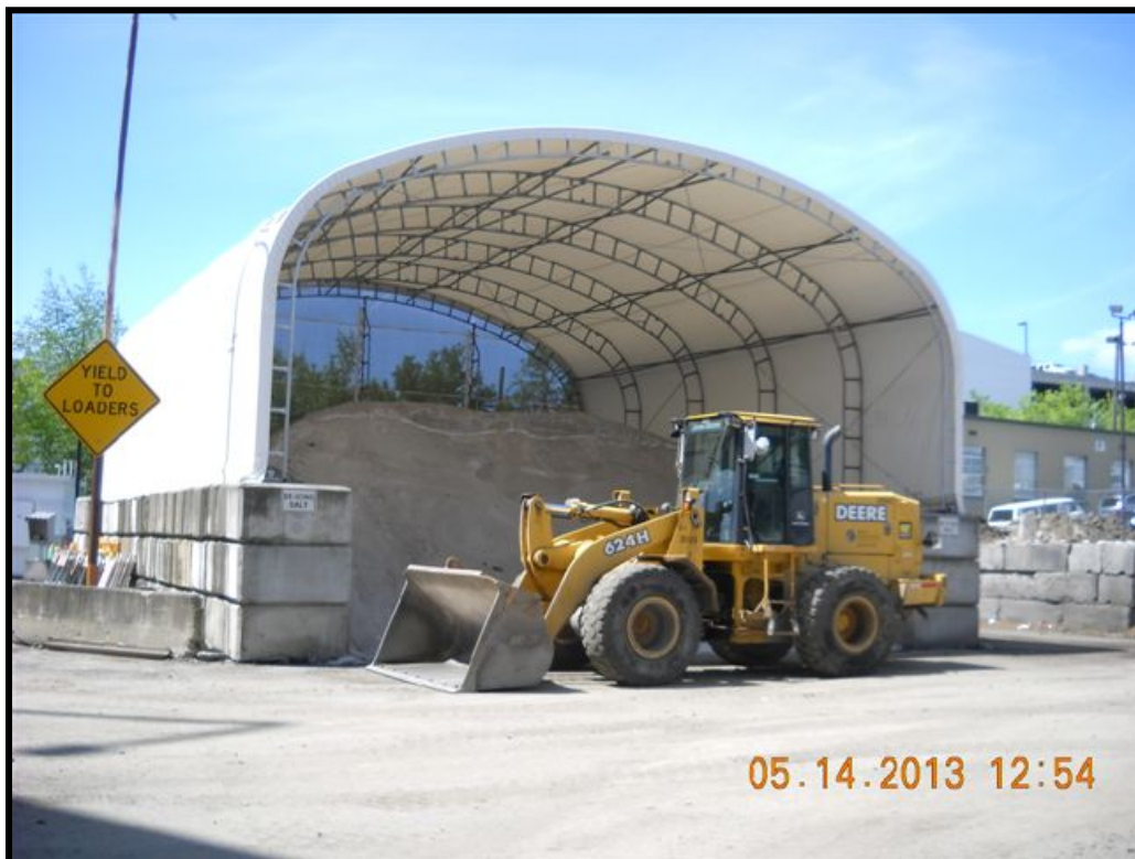
Figure 12. Covered Storage Area for Erodible Material (gravel).
