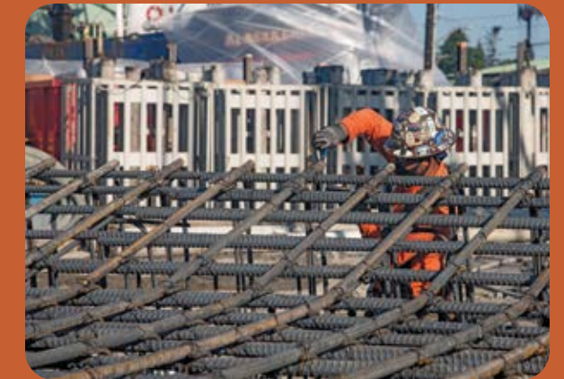
Ballard Site, Ship Canal Water Quality Project Photo Credit: Minh Carrico
