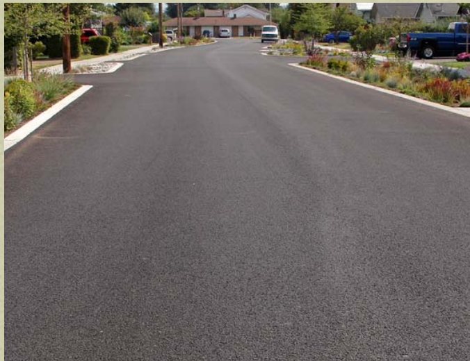
Porous Asphalt Roadway
