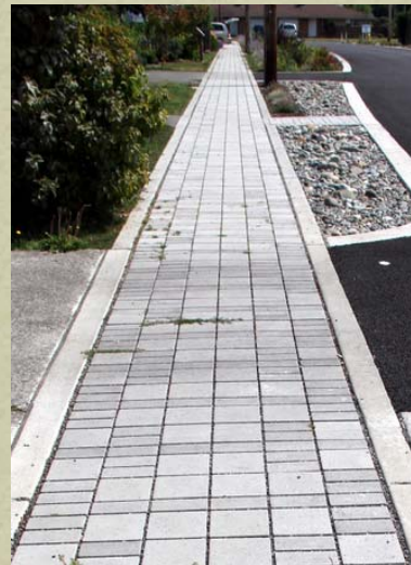
Permeable Paver Sidewalk
