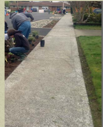
Pervious Concrete Sidewalk
