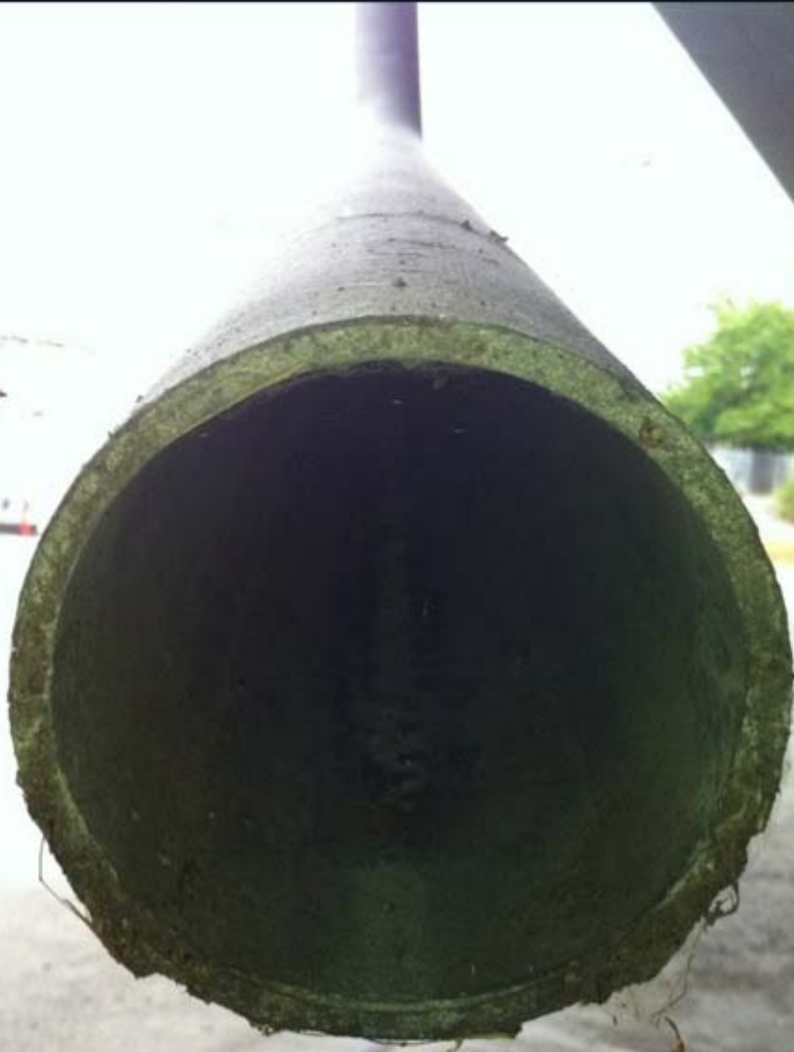
Downspout from highway
