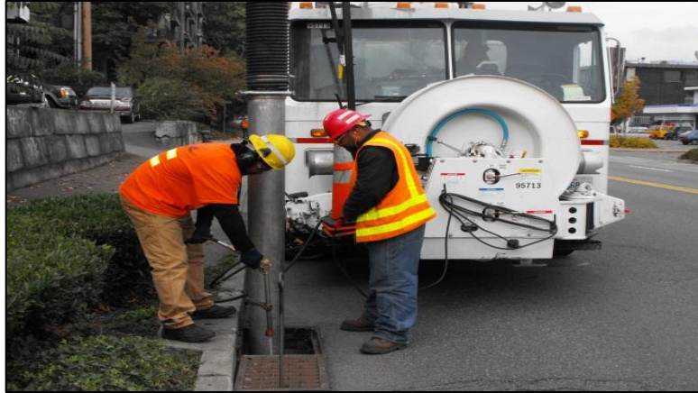
Enhanced drain cleaning
