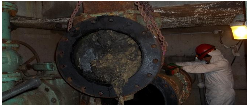
Maintenance and education to prevent SSOs due to “ragging” and FOG
