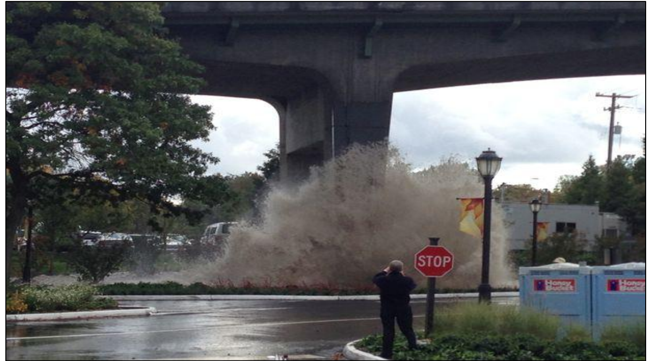
University Village water main break - 2013
