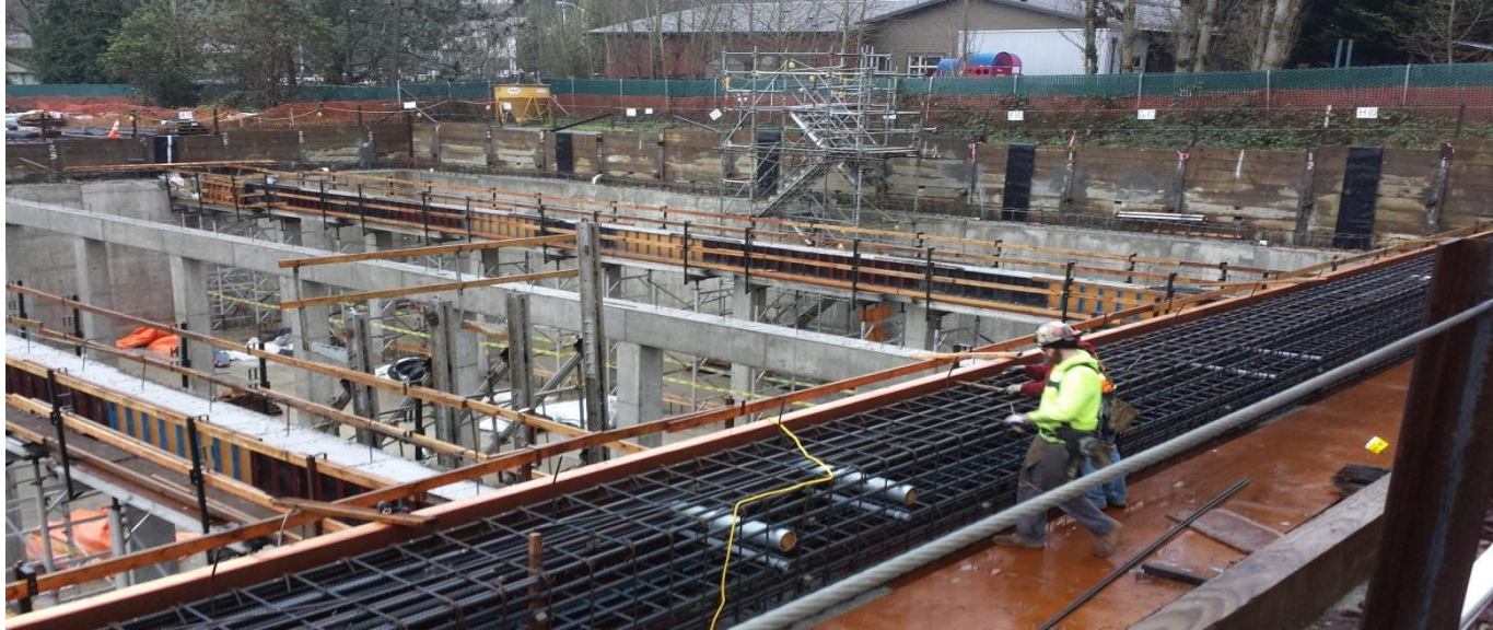
Windermere CSO storage tank
