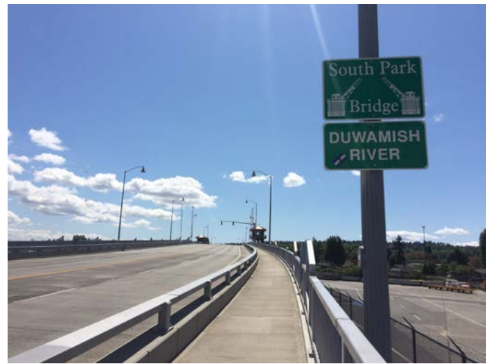
Image 1-2. South Park Bridge on 16th Ave S.
