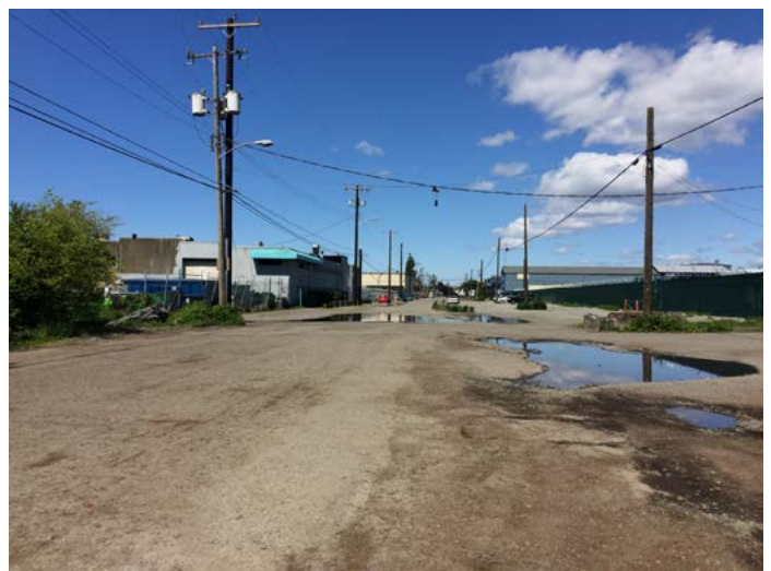
Image 1-1. View of 8th Ave S from Georgetown Pump Station Park showing puddles and lack of sidewalks.
