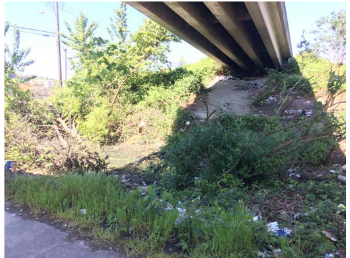
Image 1-8. Underneath WA-509 on S Front St.
