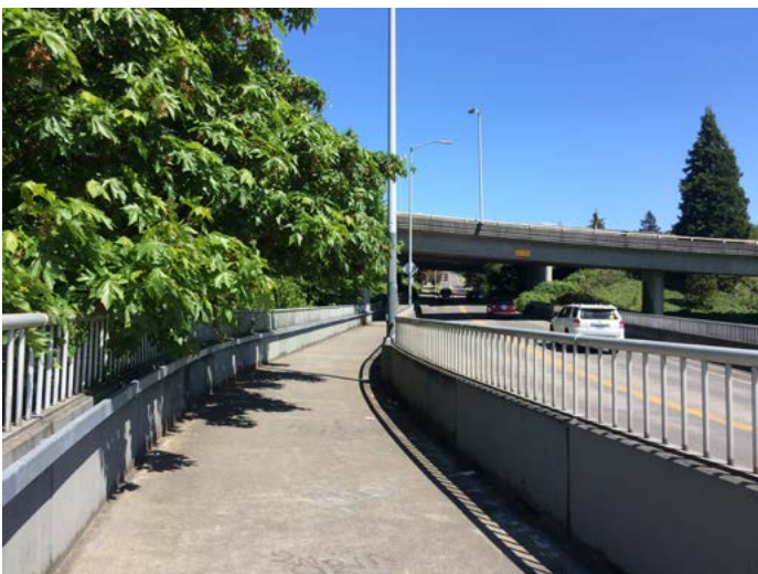
Image 1-6. Pedestrian walkway on South Lucille Street Bridge.
