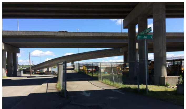
Image 1-9. Entrance to 1st Avenue South Bridge underneath WA-509 on S Front St.
