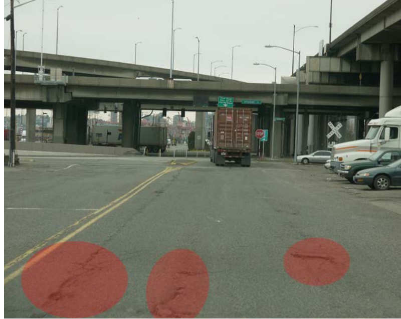
PAVEMENT RUTTING AND CRACKING ON A STUDY ROADWAY IN THE GREATER DUWAMISH MIC
