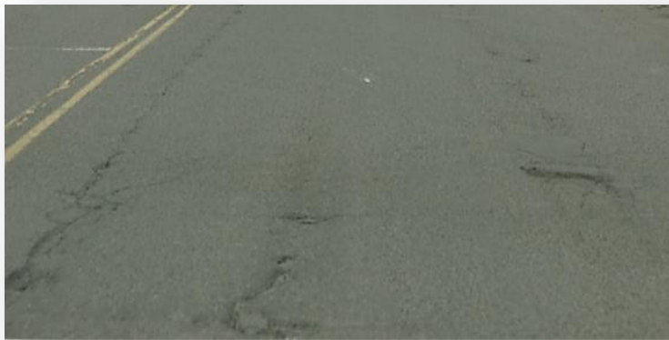
Pavement cracking and spalling. Transpo Group.
