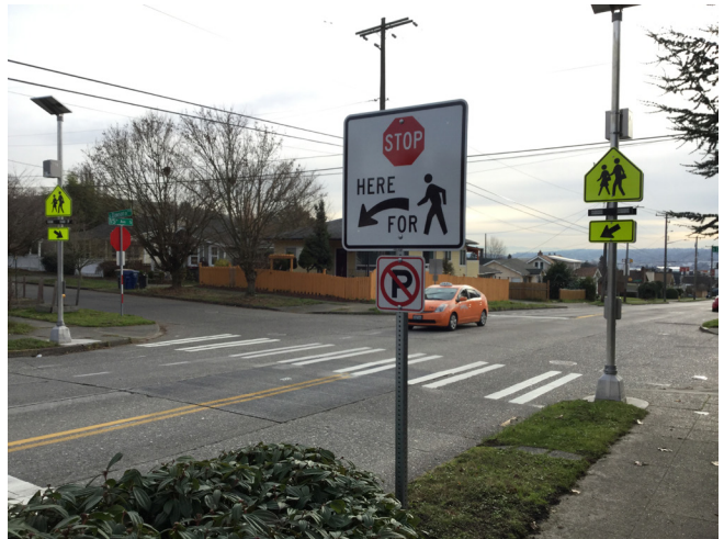
Maple ES & St George School Crossing Beacon
