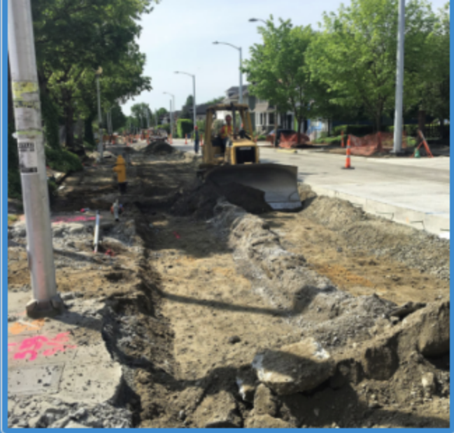
Crews removing the roadway during Phase 1 construction
