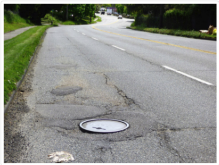
Cracked pavement on 23rd Ave S
