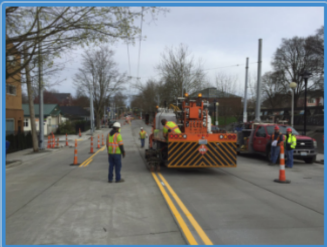
Crews restriping the new roadway in Phase 1
