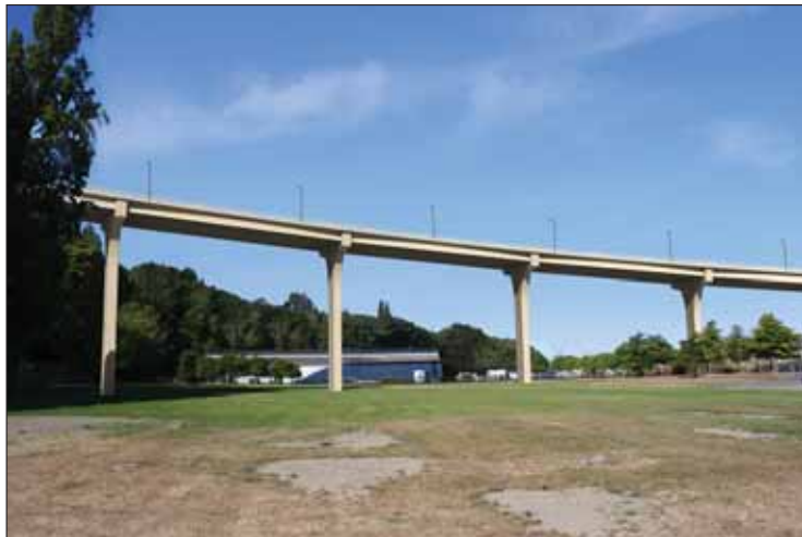
Prestressed Concrete Girders
