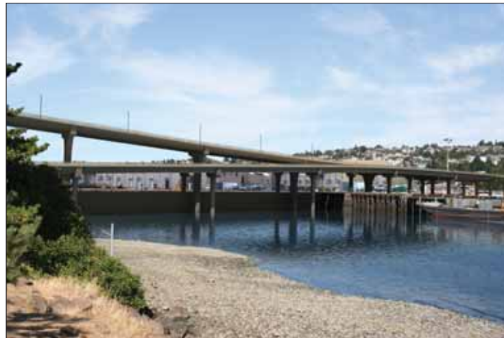
Prestressed Concrete Girders
