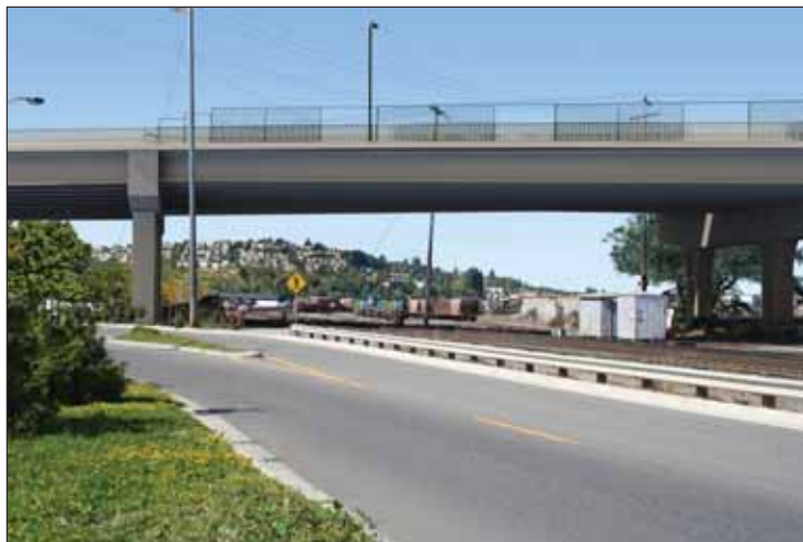
Prestressed Concrete Girders
