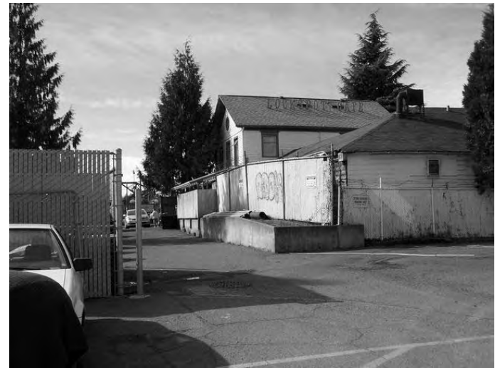
View of South and East Elevations
