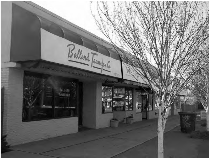
View of North Elevation
