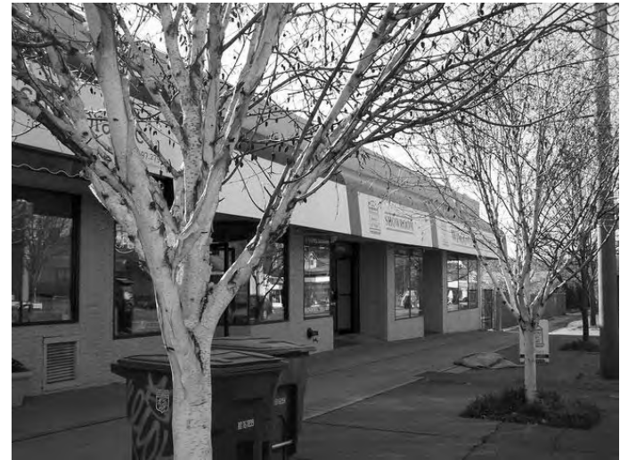
View of North Elevation
