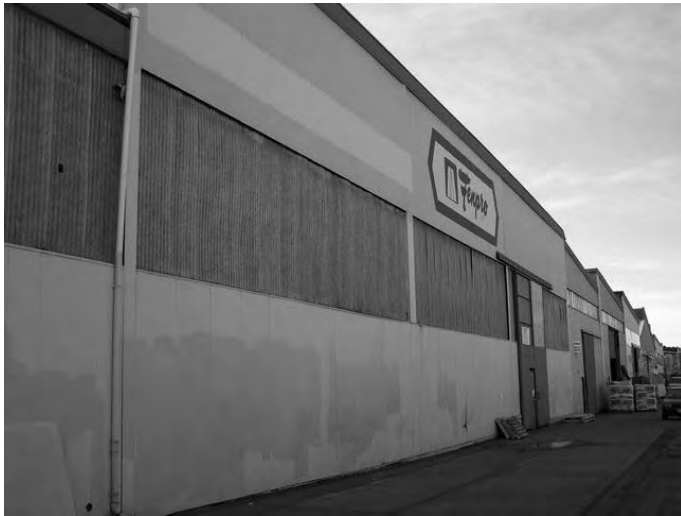
View of North Elevation
