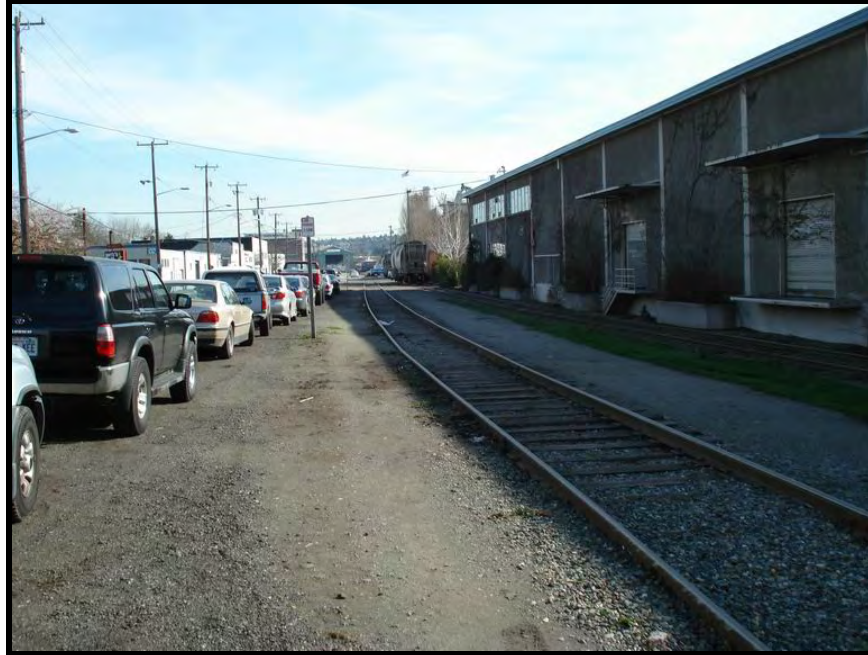
Figure 8. Area of proposed trail in Segment 2 of the Burke-Gilman Trail Extension Project (view east).
