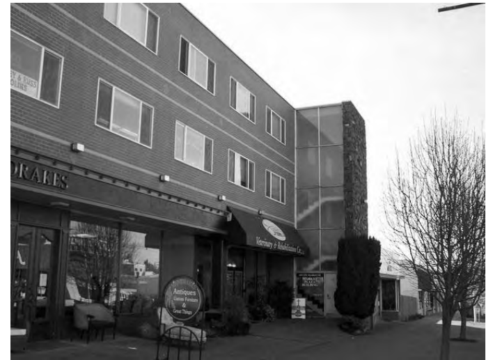
View of North Elevation
