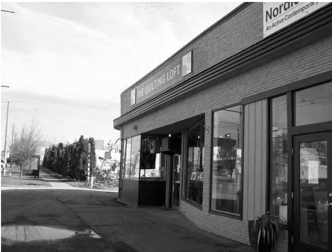
View of North Elevation
