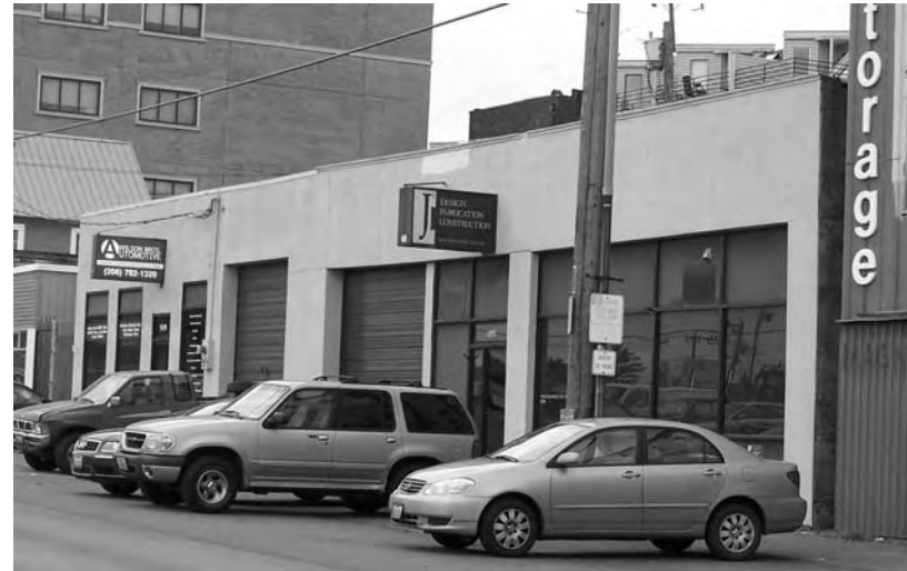
View of West Elevation
