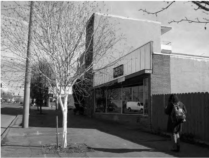
View of North Elevation
