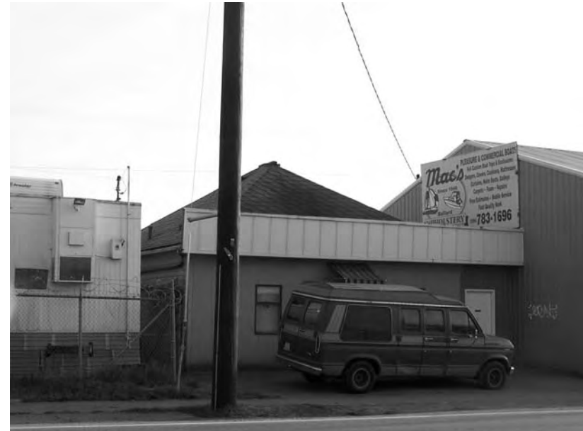
View of North Elevation
