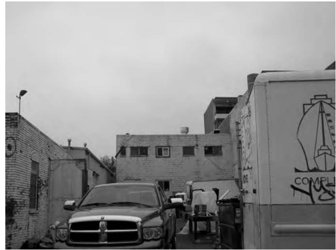
View of south elevation
