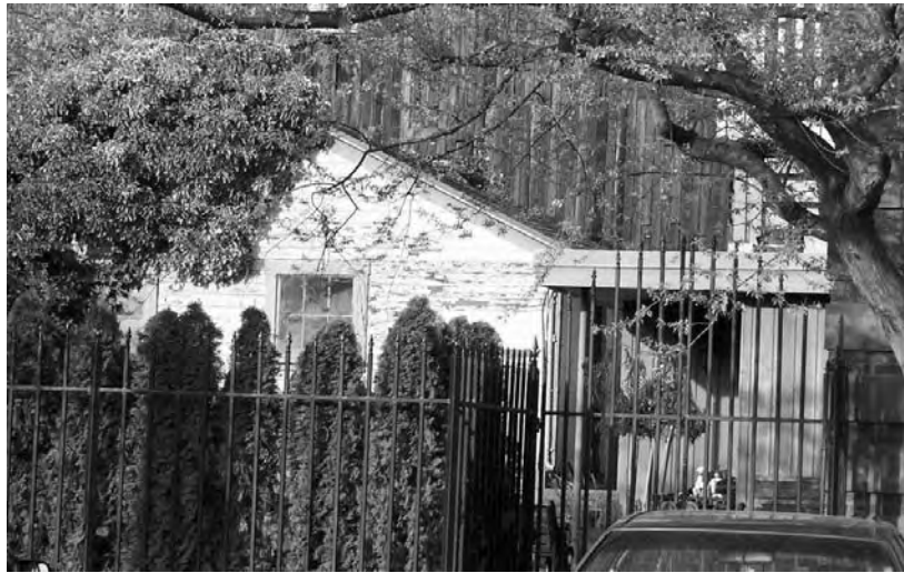
View of West Elevation
