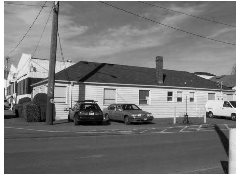
View of South Elevation taken 3/6/2007
