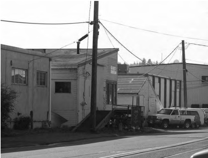
View of North Elevation
