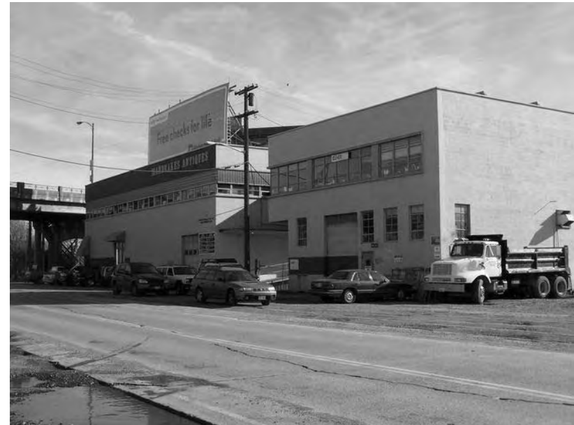
View of North Elevation
