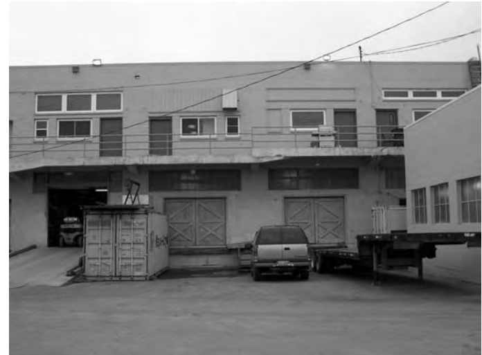
View of South elevation
