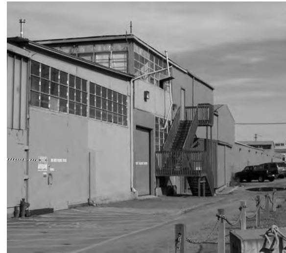
View of South Elevation
