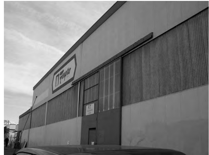
View of North Elevation
