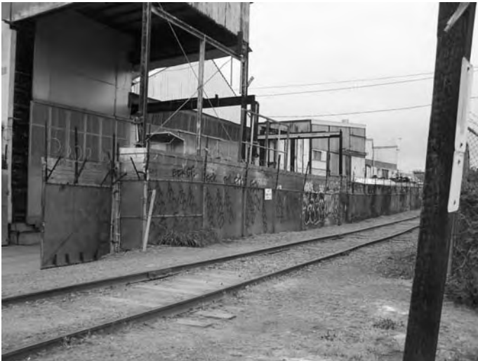
View of South elevation
