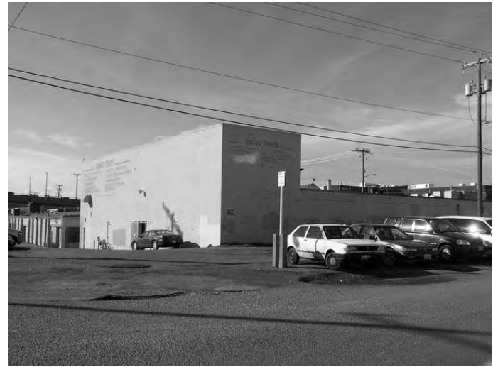
View of South and East Elevations Building #2
