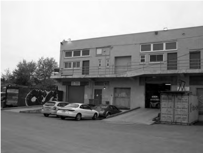
View of South elevaion
