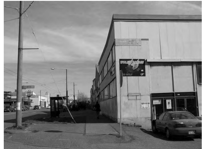
View of North and West Elevations
