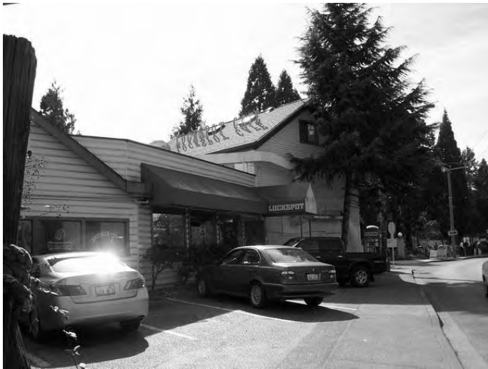
View of North Elevation
