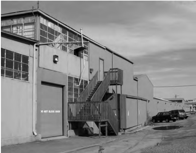
View of South Elevation
