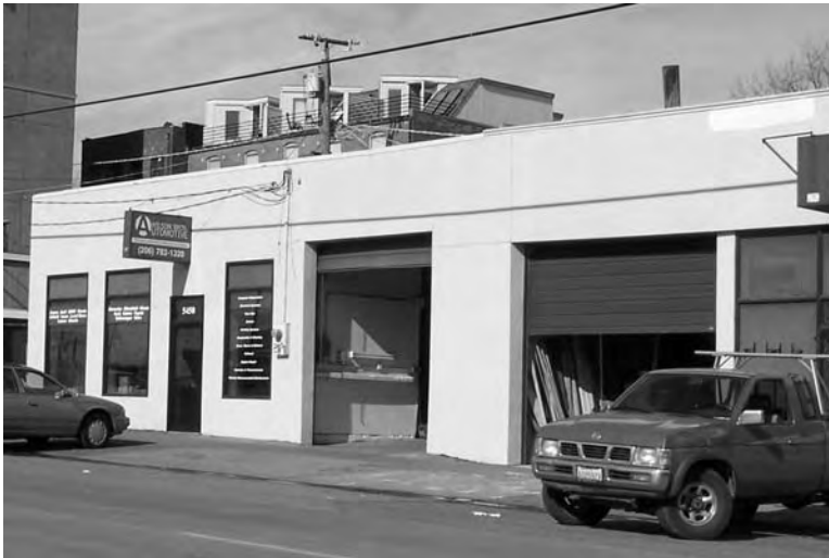
View of West Elevation
