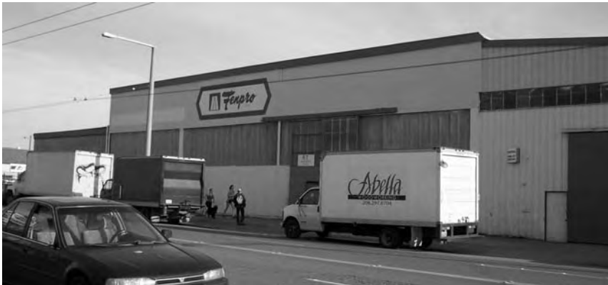
View of North Elevation
