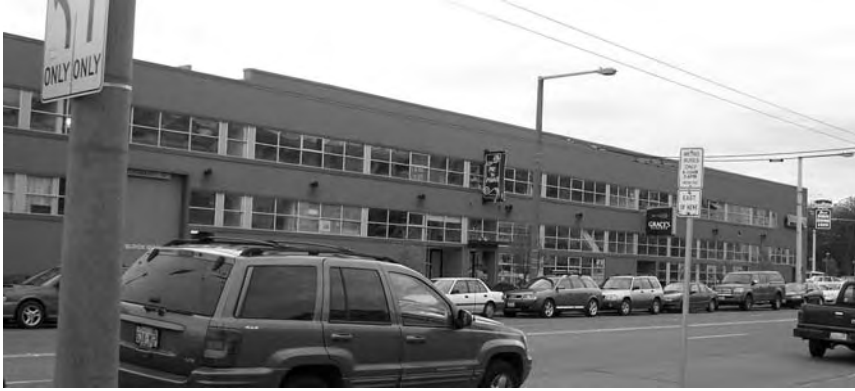
View of North Elevation
