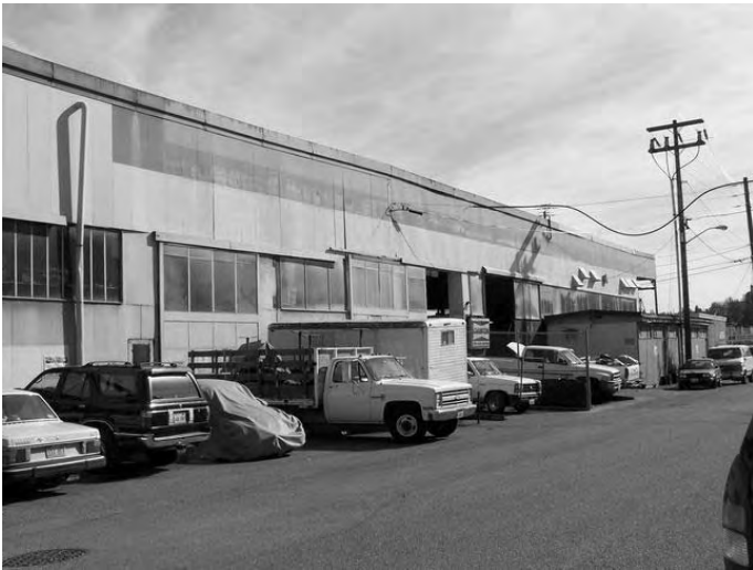
View of West Elevation
