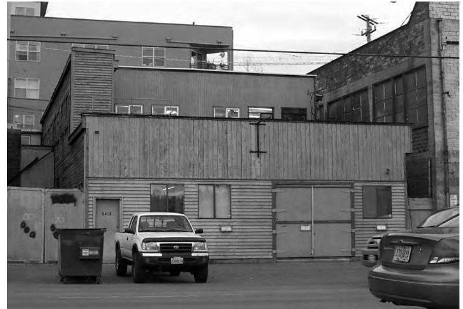
View of West Elevation
