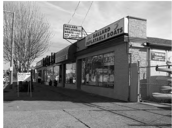
View of North Elevation
