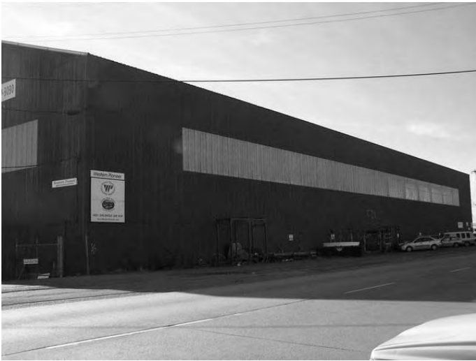
View of North Elevation
