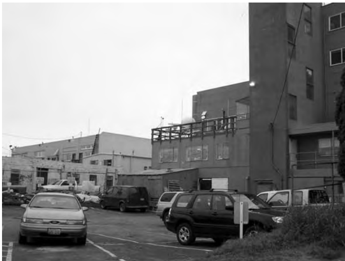
View of South elevation
