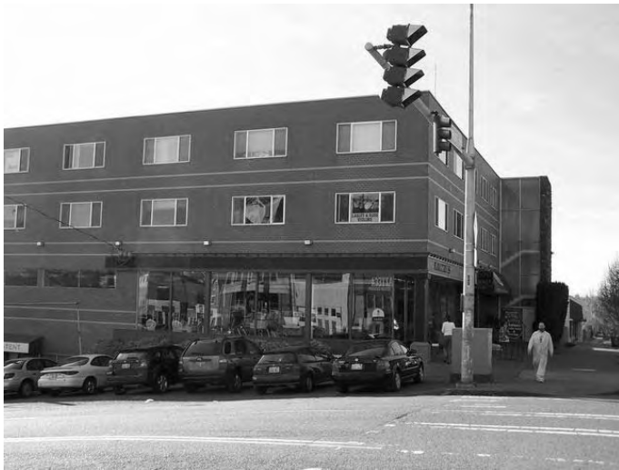
View of East Elevation
