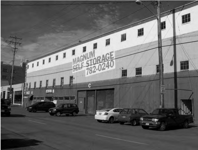
View of West Elevation
