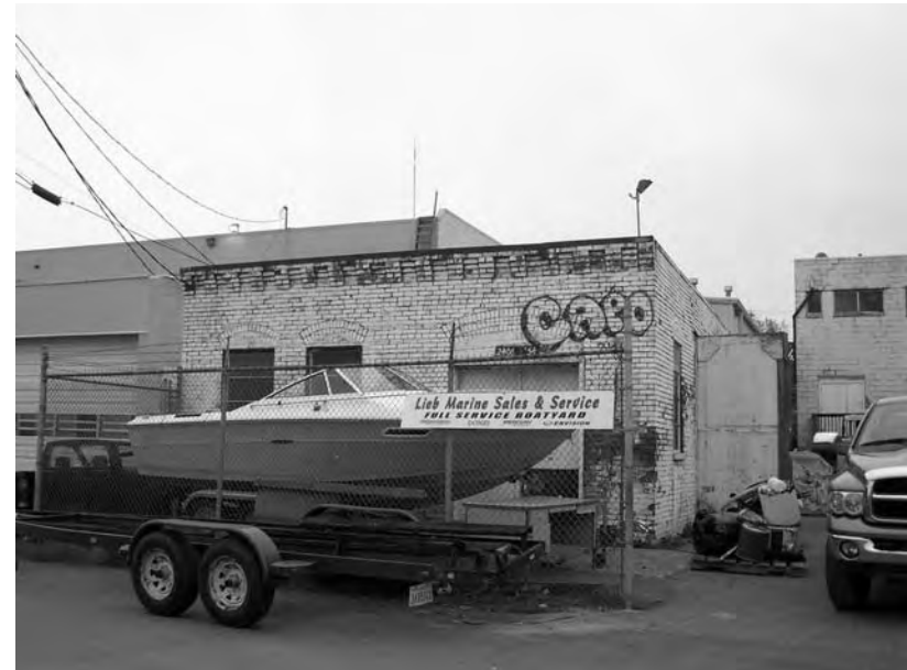
View of south elevation
