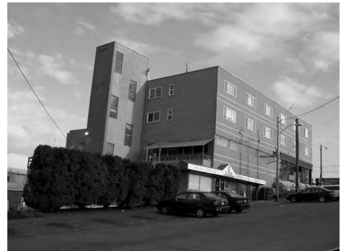
View of South and east elevations
