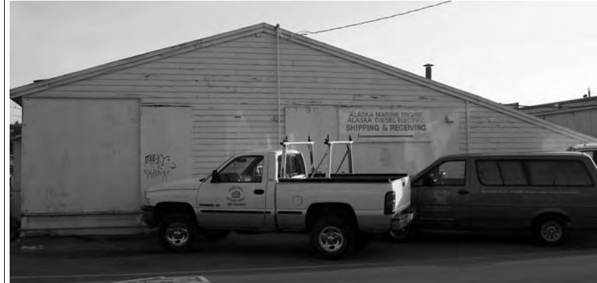
View of North Elevation
