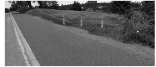
Stamped and stained asphalt sidewalk with curb (raised walkway) along NE 105th Street.
