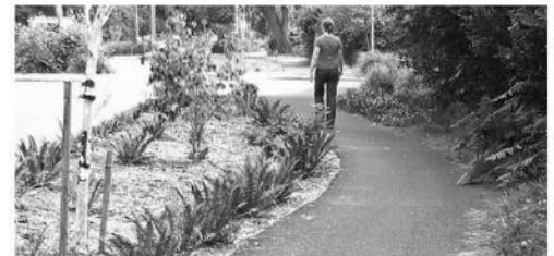
At-grade walking path behind green stormwater infrastructure without curb in the City of Shoreline.
