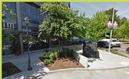
5 Enso Condominiums Denny Triangle 2201 9th Ave Green Street Improvements
