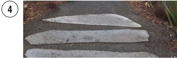
AGGREGATE PATH WITH STONE SLAB PAVERS
