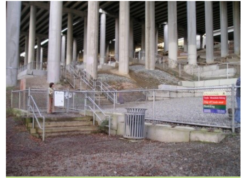
VIEW LOOKING NORTHEAST UNDER THE FREEWAY TOWARDS THE OLA
