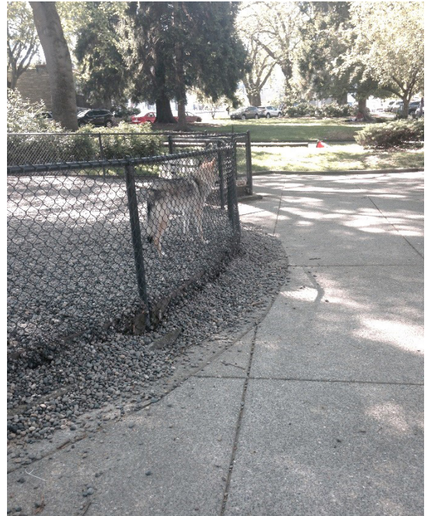
GRANOLITHIC GRAVEL SURFACING SPILLING THROUGH THE CHAIN LINK FENCING AT DENNY PARK
