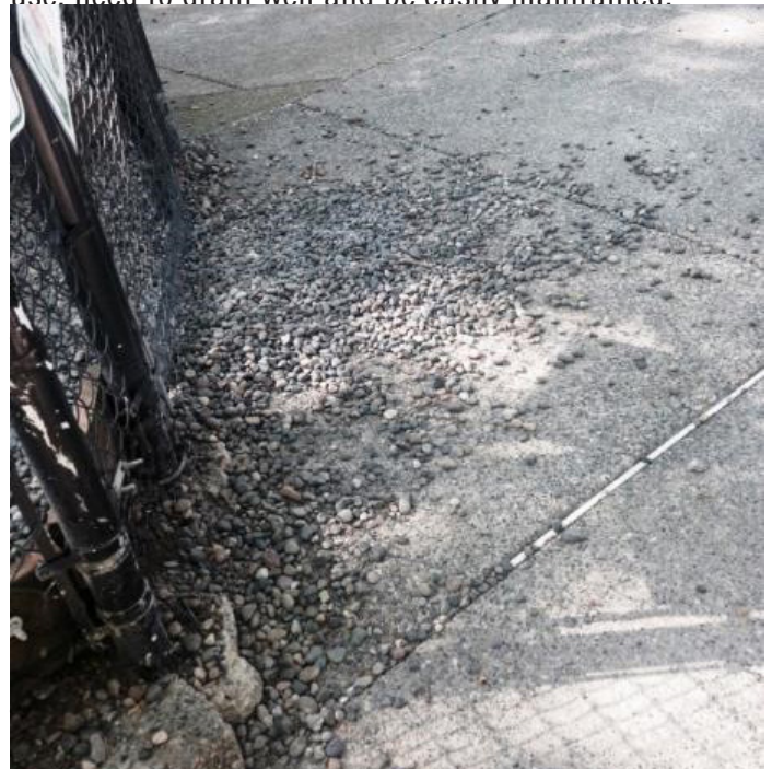
GRANOLITHIC ROCK SURFACING AT DENNY PARK
