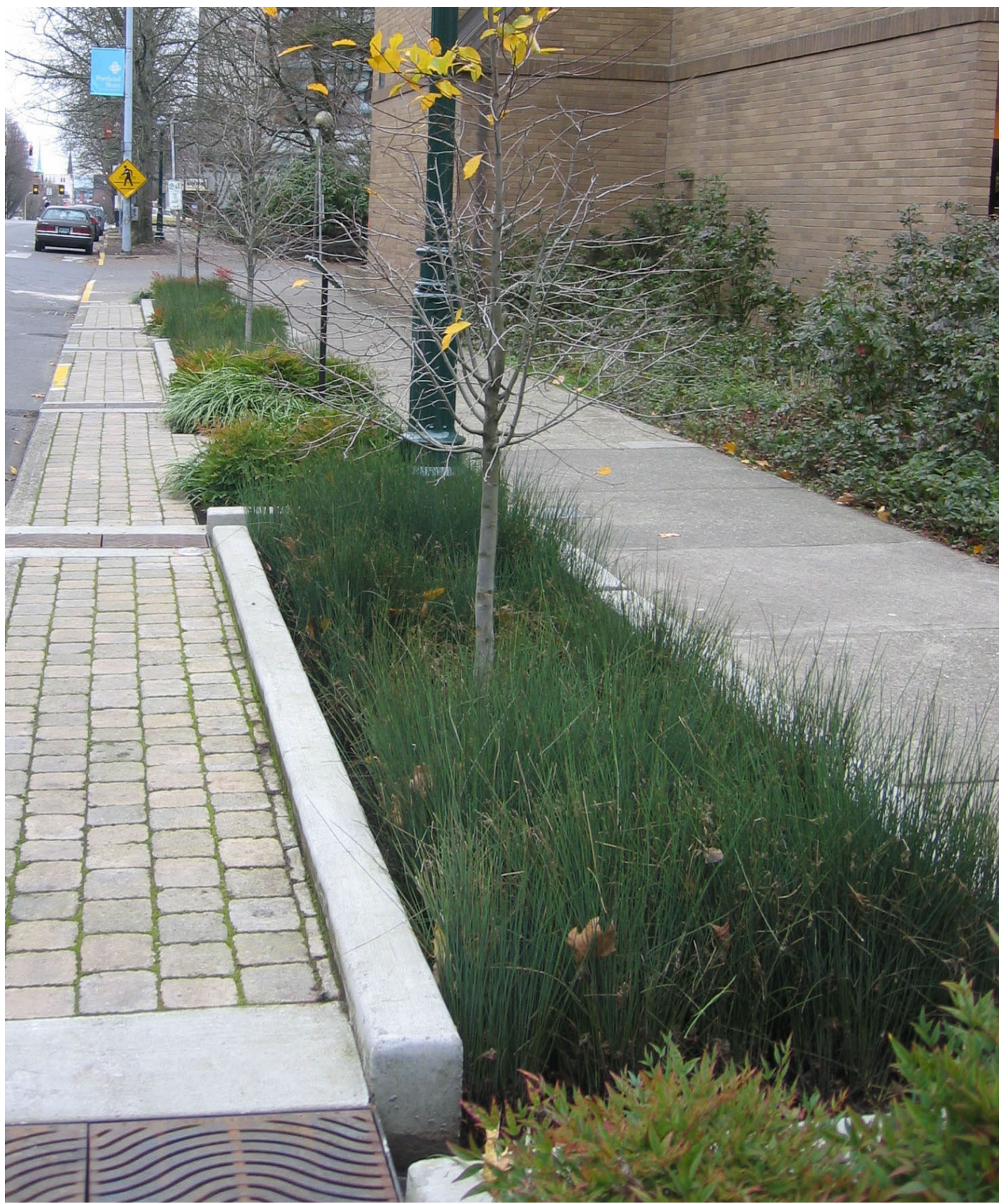
Stormwater planters in Portland
