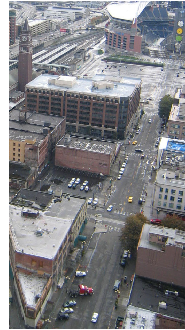
Existing Conditions- View from Smith Tower
