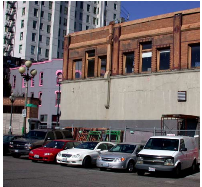
Building under renovation near Second Avenue and Washington
