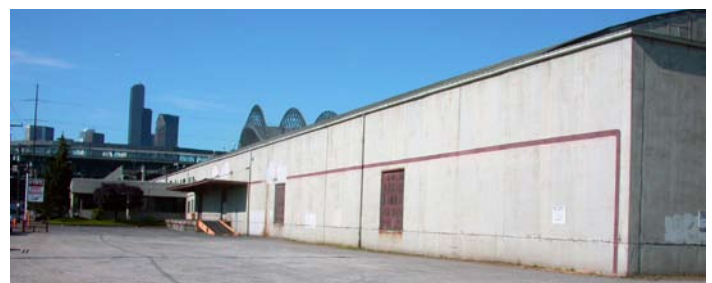
Warehouse at Occidental Avenue, near Holgate Street
