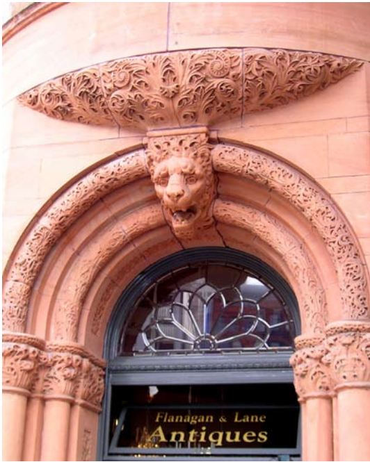
Interurban Building detail
