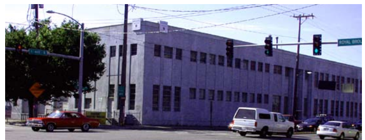
Building at First Avenue S. and Royal Brougham Way
