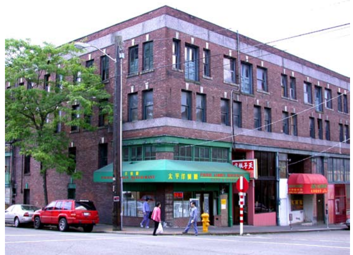
East Kong Yick Building
