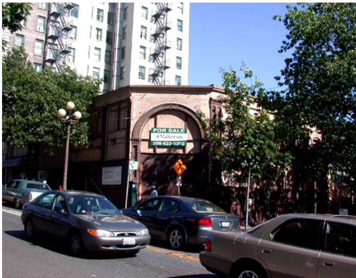
Campbell-Fuller Building, at Second Avenue and Yesler Way
