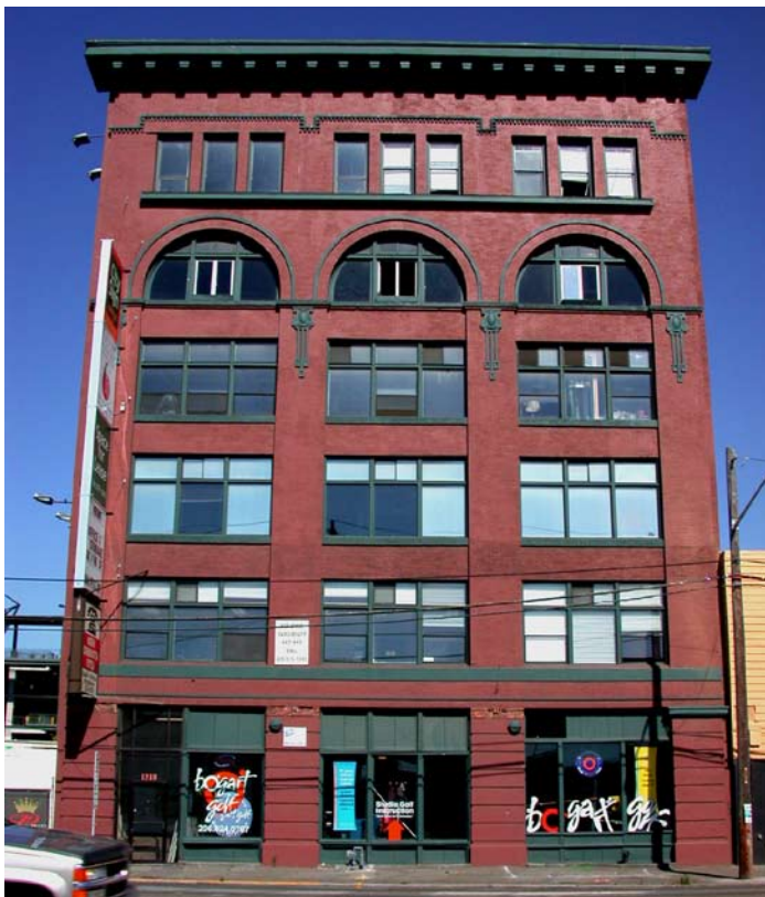
Brick building on First Avenue
