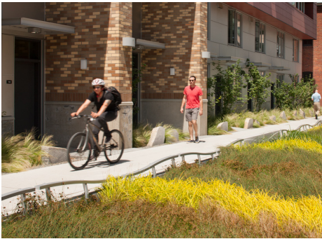
This Swale provides for storm water runoff enhances the streetscape in the Cascade neighborhood.
