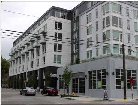
Context - light industrial building design; pilasters, large casement windows, brick and terra-cotta cladding.
