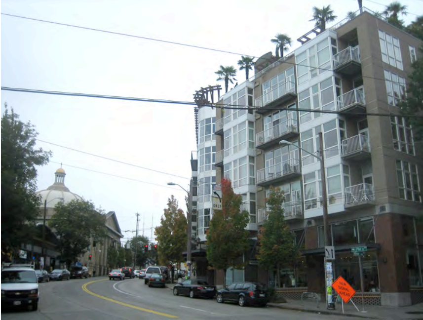
The rooftop palm trees of the Pike Lofts are visible from the street below, and from a distance, and are identifying elements of the building.
