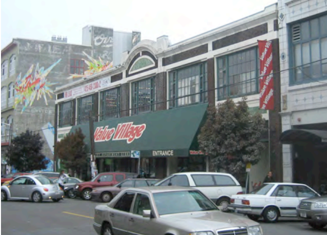
Value Village on Eleventh Avenue: The awning is too large, and obscures a view of the storefront.
