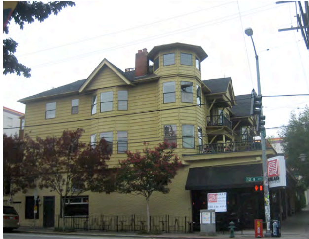
Northeast corner, 12 th Avenue and Pike Street.
