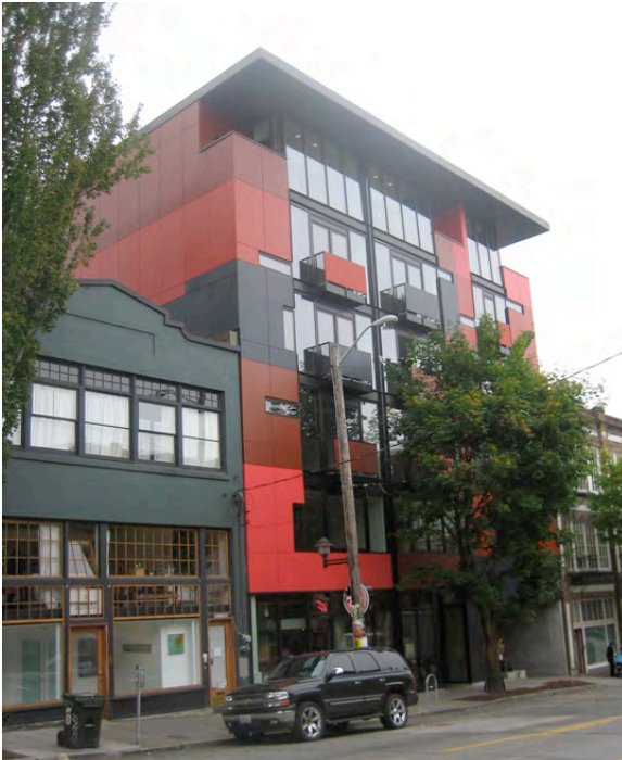
Balconies on 1111 East Pike Street.
