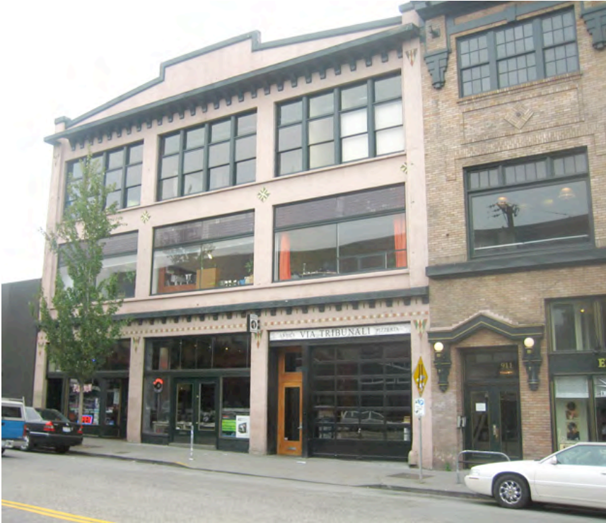
South side of Pike Street between Broadway and Tenth Avenue: Cornices and parapets are common elements in older commercial buildings.
