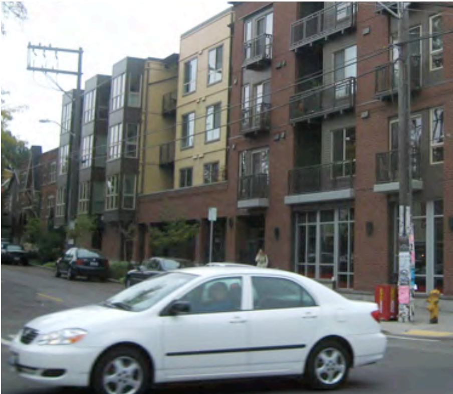
Parking garage entry for the Braeburn is located on 14 th Avenue.
