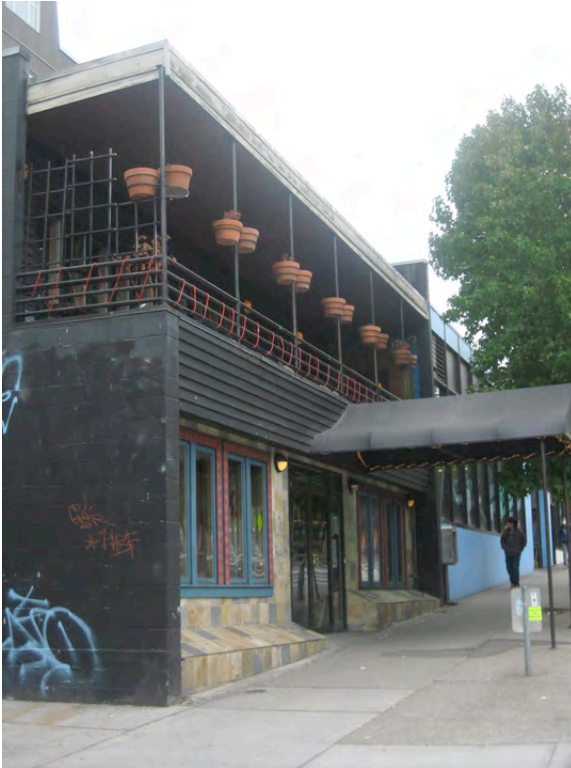
North side of Pine Street, near Crawford Place: the building entry is flush to the sidewalk, scaled for pedestrian access, placed in the center of the building, marked by exterior lamps, and covered by a canopy.
