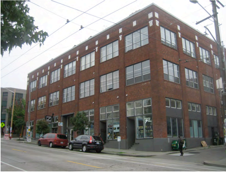
South side of Pine Street, at Crawford Place.
