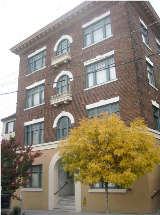
East side of Melrose Avenue between Pine and Pike Streets: Smaller bays, contrasting trim color give this residential building a smaller scale than the commercial structures around the corner.
