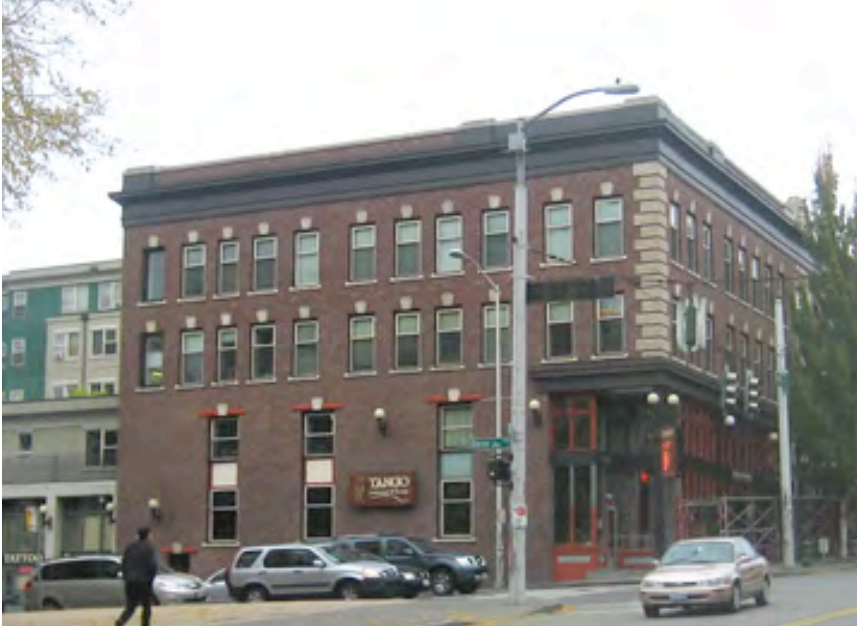
Northeast corner of Boren Avenue and Pike Street.
