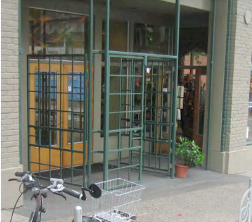
South side of East Pine Street at Summit Avenue: An ornamental gate that remains open during business hours and is locked at night.
