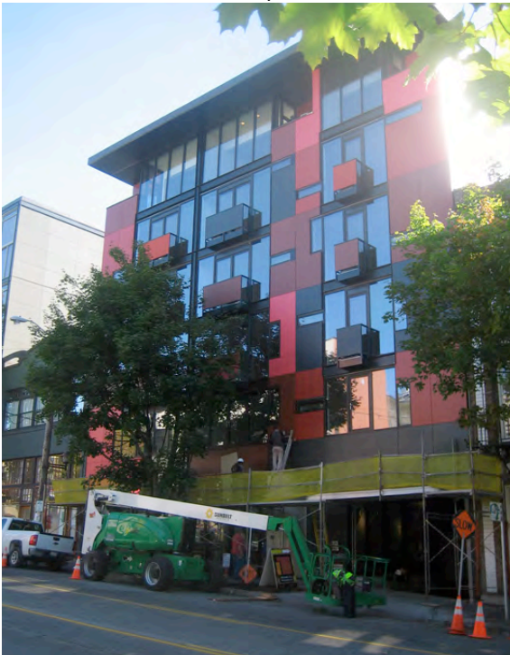
Sturdy materials that evoke industrial use, strong vertical elements, large expanses of glass, and a cornice line are some of the elements these two new developments (1111 East Pike and Agnes Lofts) have in common with the older character buildings in Pike-Pine.
