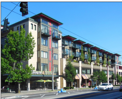
Setbacks, modulation and changes in material all contribute to making the scale of this large structure compatible with the established development context.
