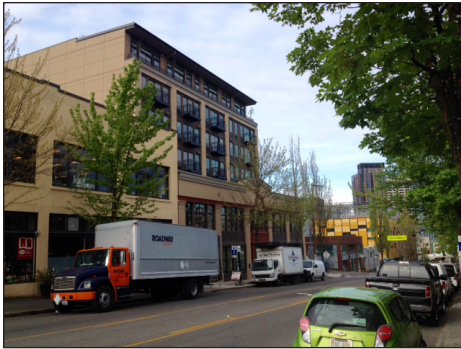
Elements of historic character structure reflected in a subtle way in the transition from the original building to the new structure above.
