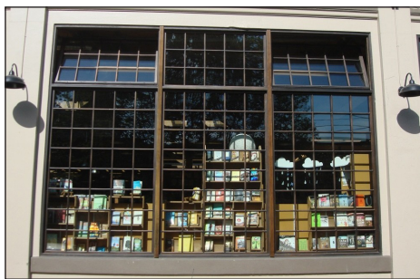
Window trim detailing.
