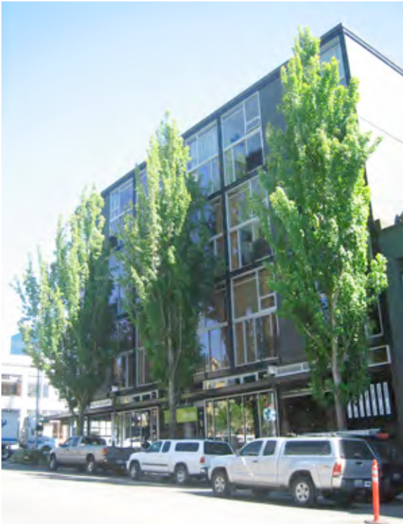
Expansive glazing and rhythmic structural frame of the Agnes Lofts.
