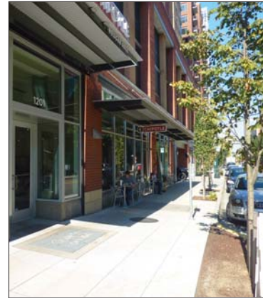
Retail with weather protection for pedestrians.
