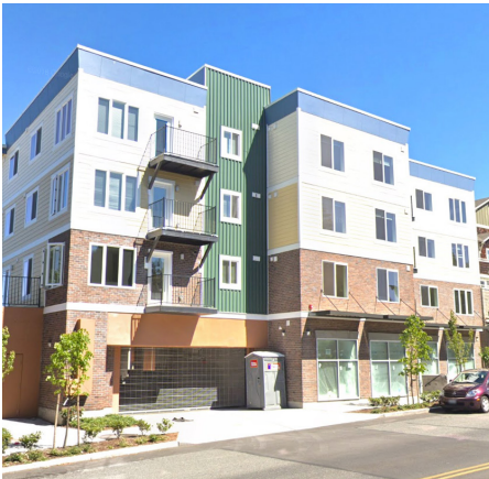
Multifamily housing development on 15th Ave NE
