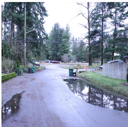
Example of ponding issues in the Station Area
