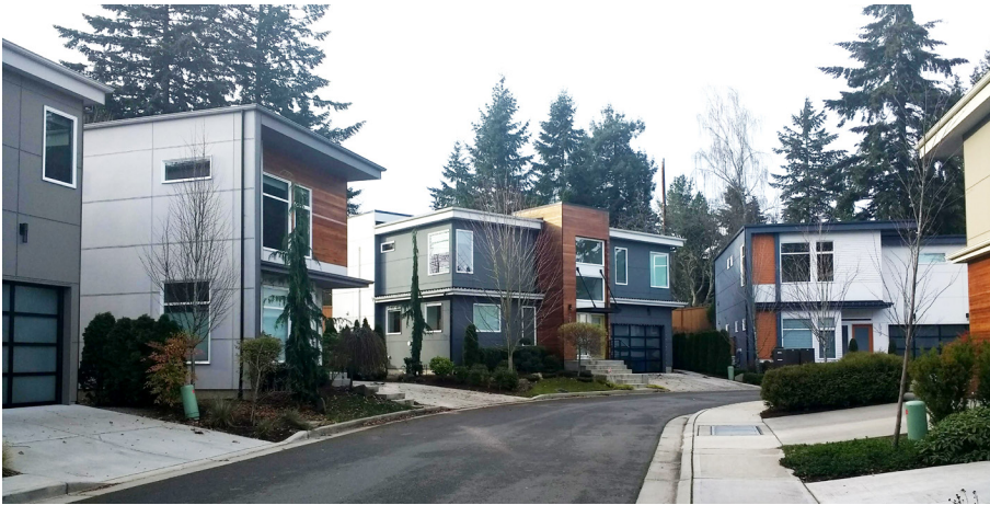
Single family housing development at Meridian Ave N and Roosevelt Way N
