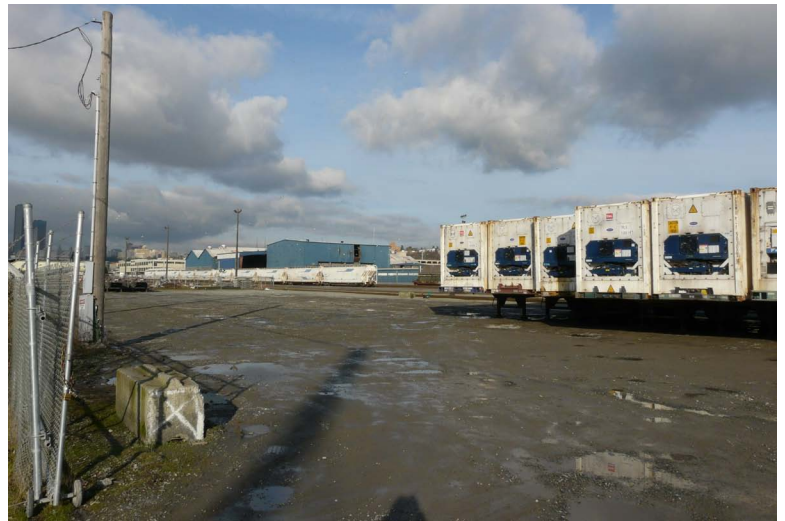
Outdoor storage is very common in the Duwamish. This might give one the impression that large areas of land are vacant. Buildings are low and small compared to their lots, the average FAR of industrial uses in the Duwamish is .32
