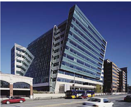
505 Union Station responds directly to the adjacent transit center.
