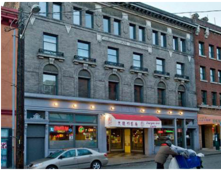
Typical facade articulation in Chinatown
