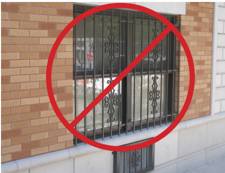
Prohibited bars installed on the building facade
