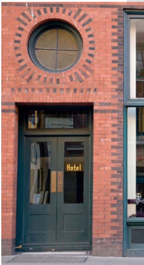
Existing building in the ISRD
