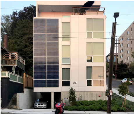
Solar panels add interest to facade and help meet the buildings energy needs.
