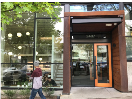
This north-facing live/work unit uses a high level of transparency to enliven the street edge and connect the indoor and outdoor environments.
