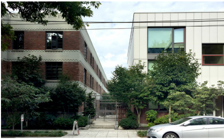
New construction mimic the scale and massing of the existing streetscape while using contemporary materials and window patterns.
