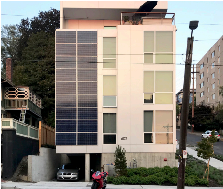
Solar panels add interest to this facade and help meet the buildings energy needs.
