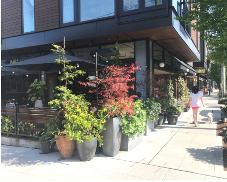
This building uses a structural building overhang over a voluntary setback and retractable canopies to provide weather protection over a narrow sidewalk condition.
