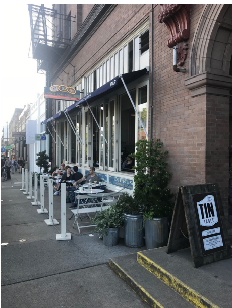
Cafe uses operable windows and retractable sun shades to provide shading and natural cooling, as well as overhead weather protection when needed.
