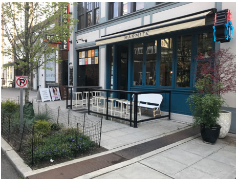
Small scale retail facade fits into the overall building concept and allows for personalization with color, signage and retractable canopy.
