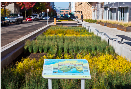
Interpretive signage explaining “green stormwater infrastructure.”
