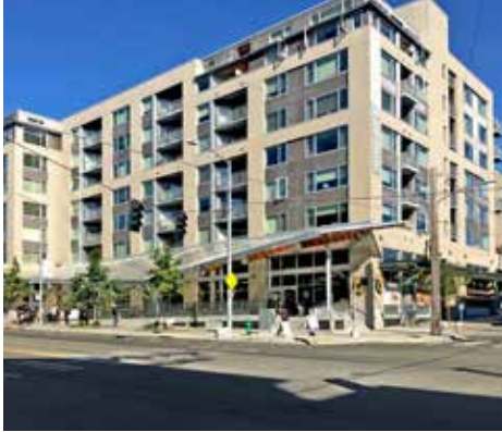
The Ballard Public Lofts is a positive example of a six-story mixed-use building that is a good fit for both the Character Core and General Commercial Character Districts.
