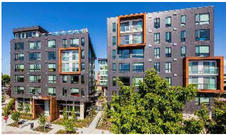
New buildings in the Character Core bring different architectural styles, but maintain strong presence and detailing.
