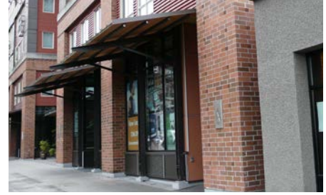
An example of first floor retail in a multifamily building on NW Market St.
