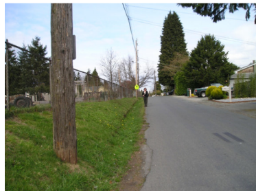
Ditch & fence along 13th Ave.
