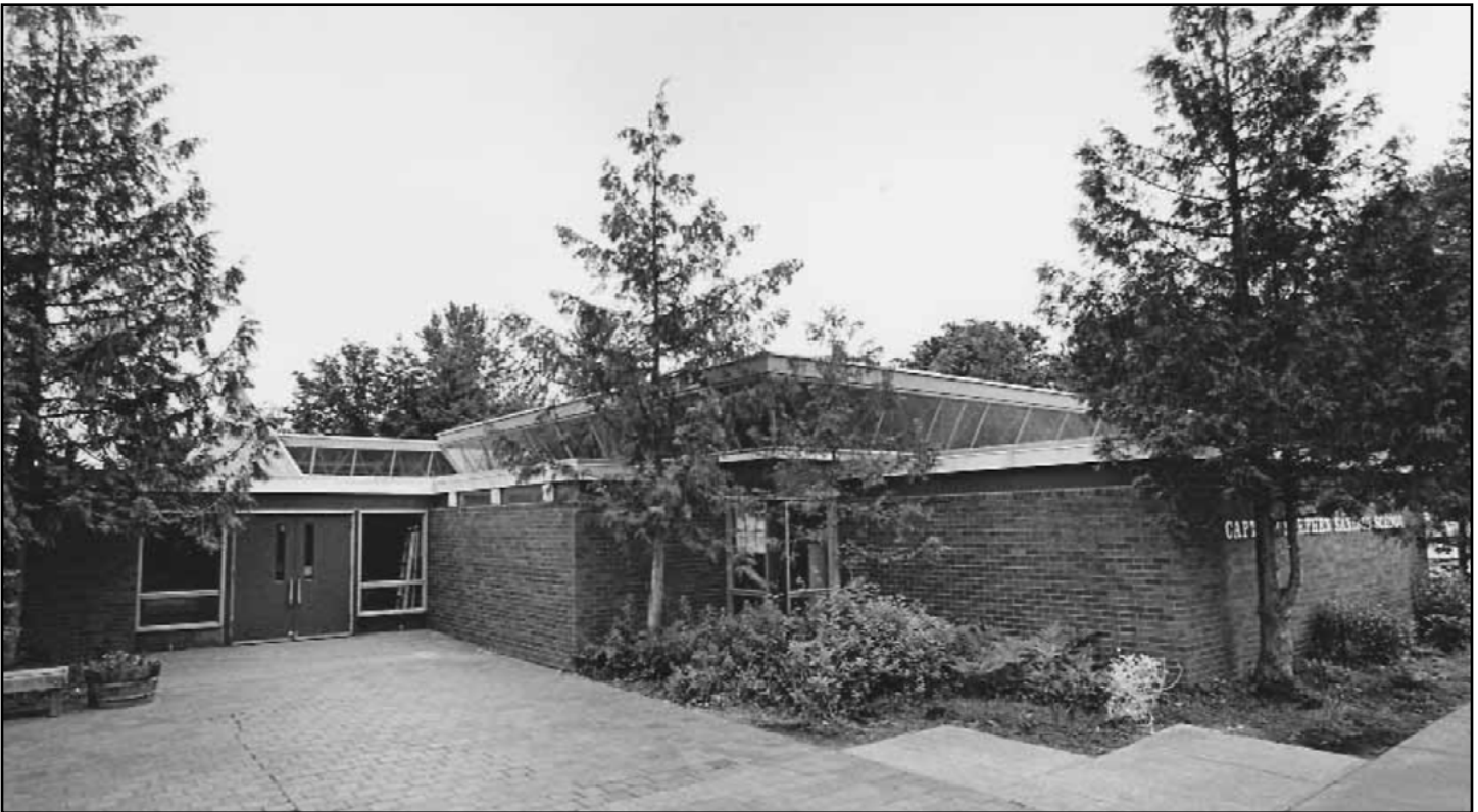
Figure 20. Captain Steven E. Sanislo School (Sullam, Smith & Associates, 1970)
