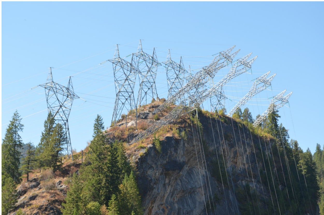
Photo 23 of 25: (WA_PendOreille_BoundaryDam__023) Boundary Dam Transmission Line, Pickleforks, camera looking NW from dam crest (A)
