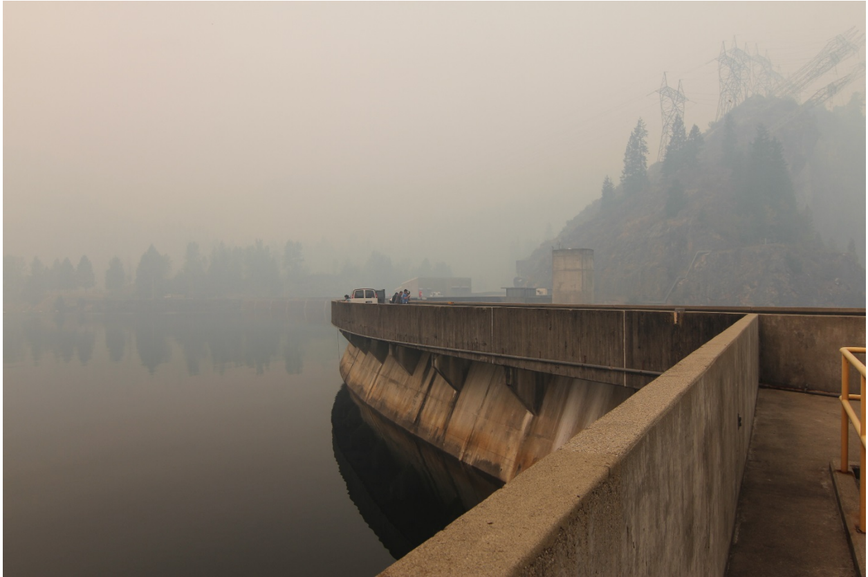
Photo 10 of 25: (WA_PendOreille_BoundaryDam__0010) Boundary Dam, Dam Crest, camera looking W, toward Forebay (K)
