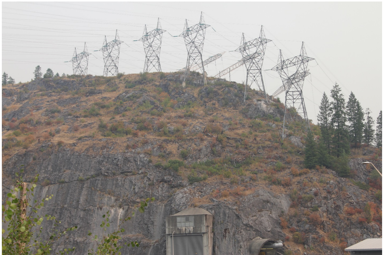
Photo 22 of 25: (WA_PendOreille_BoundaryDam__022) Boundary Dam Transmission Line, camera looking N from Forebay (K)
