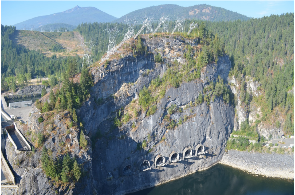
Photo 8 of 25: (WA_PendOreille_BoundaryDam__008) Boundary Dam, Powerhouse formation (Left Abutment), showing Transformer Bays, Transmission Line, camera facing West, from Vista House Overlook (A)
