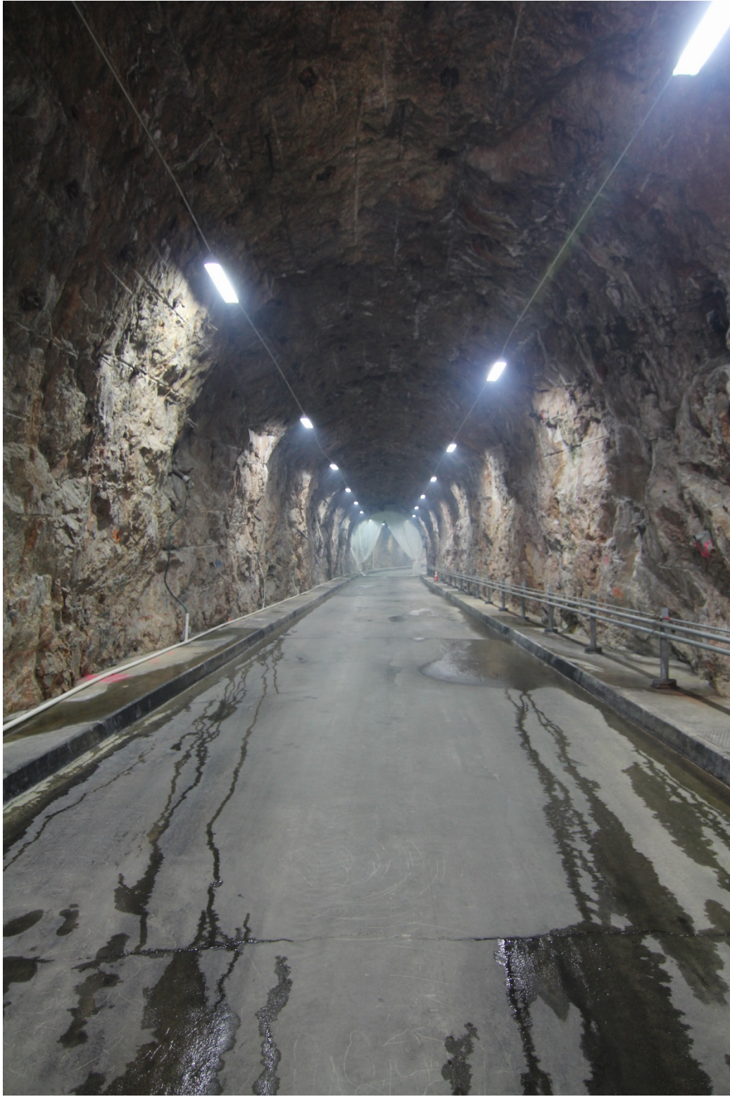
Photo 12 of 25: (WA_PendOreille_BoundaryDam__012) INTERIOR: Dam Access Tunnel, camera looking SE from near entry (K)
