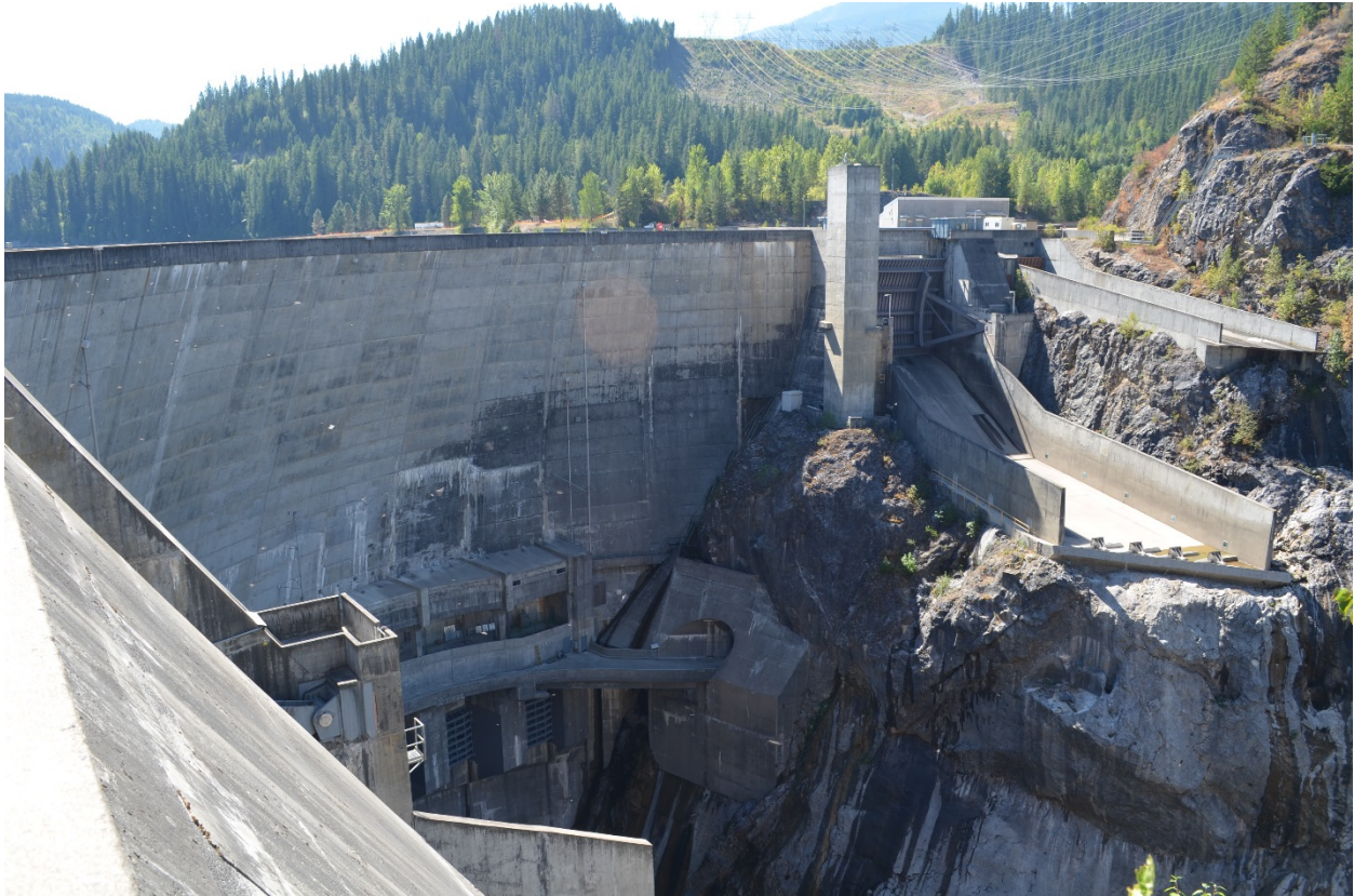
Photo 6 of 25: (WA_PendOreille_BoundaryDam_006) Boundary Dam, Left Spillway, Sluice Gates on downstream face, camera facing SW from dam crest at right abutment (A)
