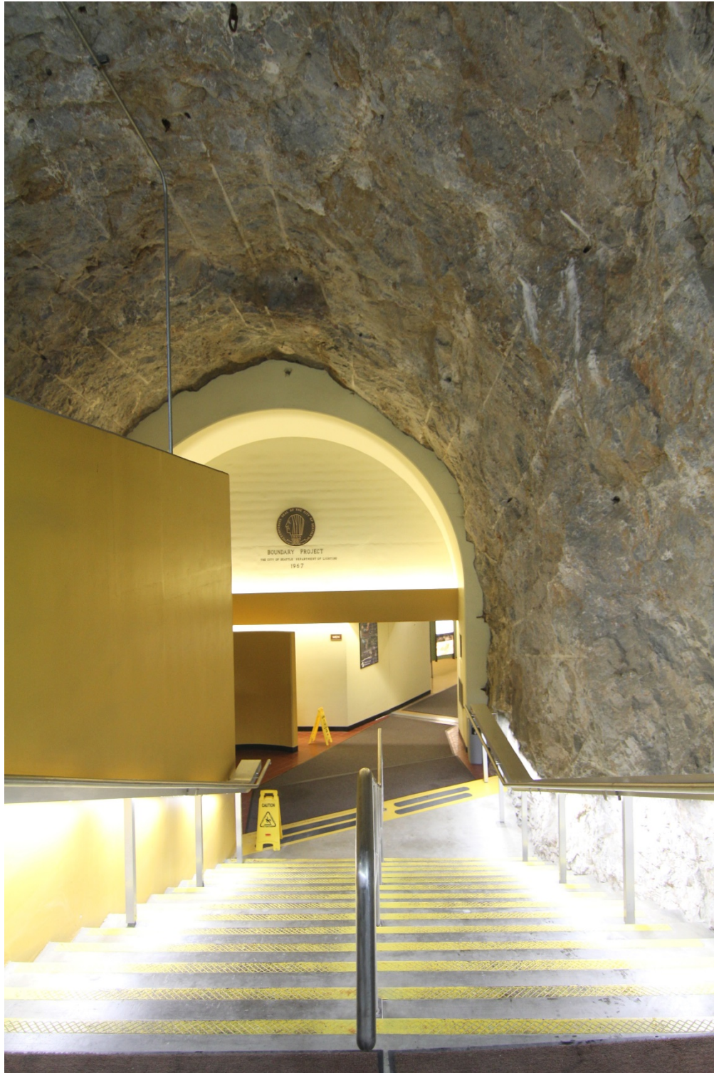
Photo 13 of 25: (WA_PendOreille_BoundaryDam__013) INTERIOR: Visitors' Gallery Entryway, from Powerhouse Access Tunnel, camera looking W (K)
