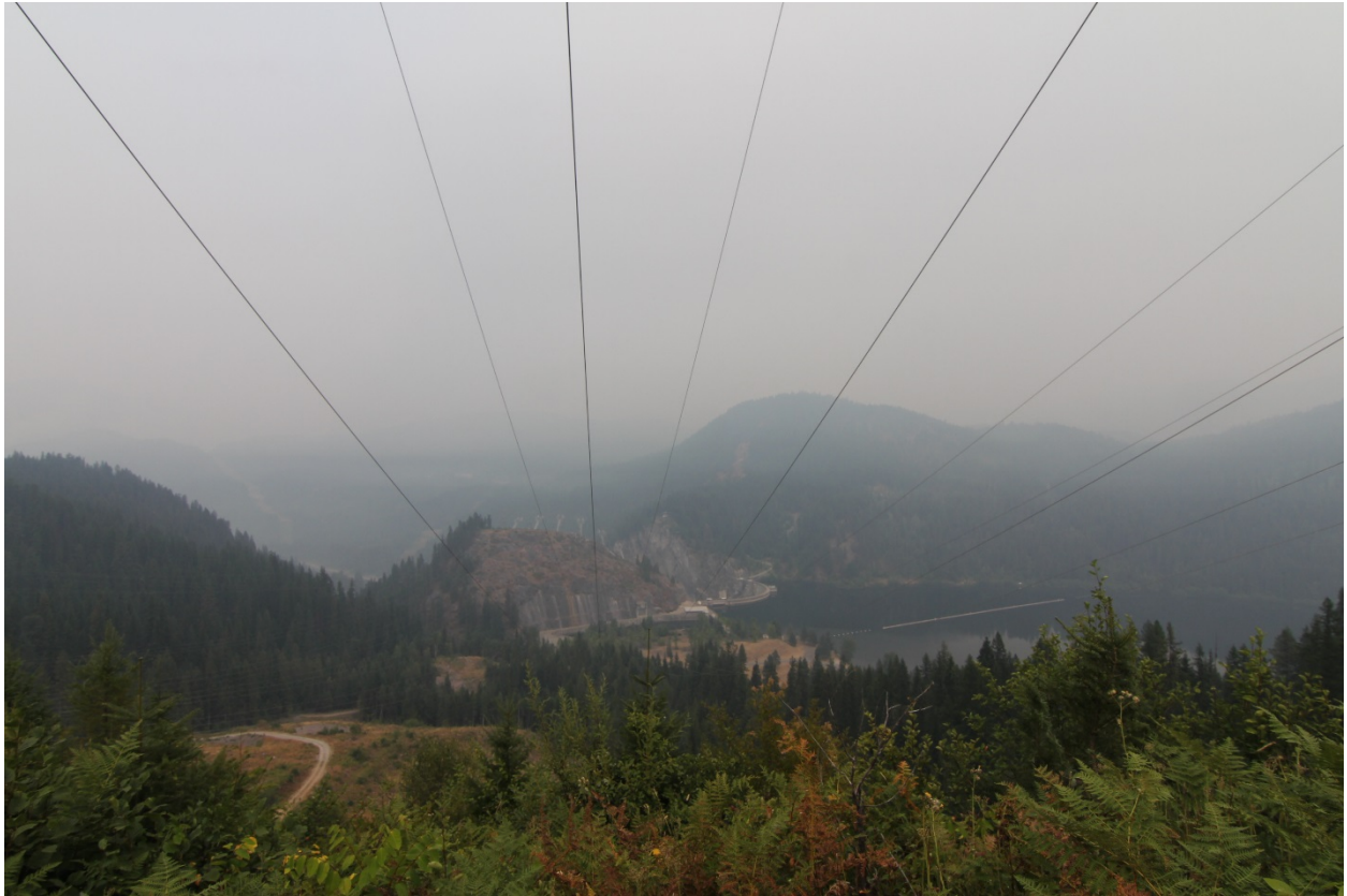
Photo 24 of 25: (WA_PendOreille_BoundaryDam__024) Boundary Dam Transmission Line and project overview, camera looking NE from BPA Boundary Substation, toward dam and powerhouse (K)
