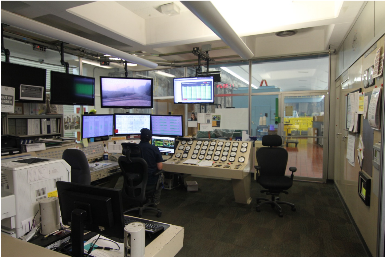
Photo 16 of 25: (WA_PendOreille_BoundaryDam__016) INTERIOR: Boundary Powerhouse Control Room, camera-looking E, toward main floor of the Machine Hall (K)
