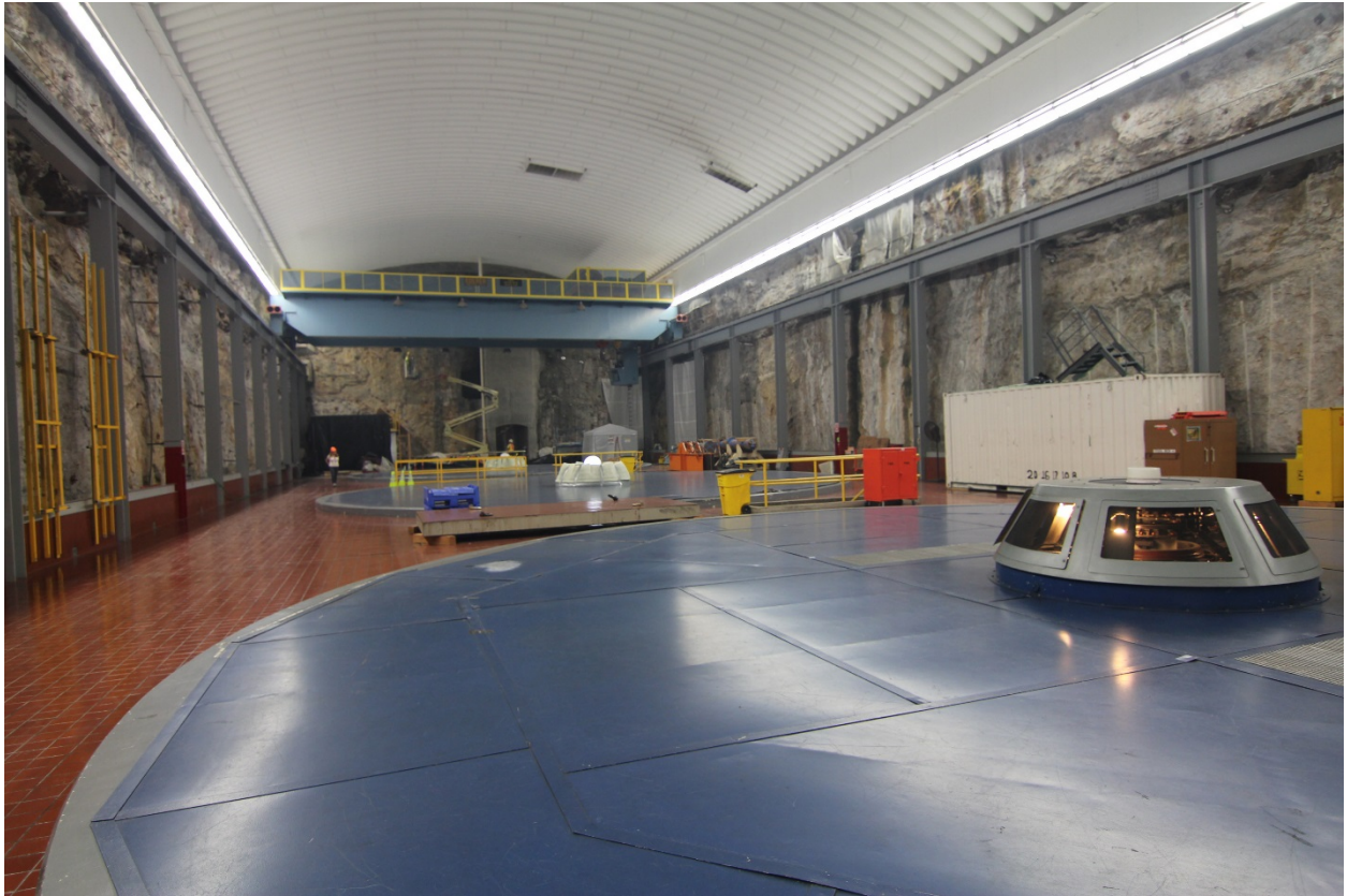
Photo 15 of 25: (WA_PendOreille_BoundaryDam__015) INTERIOR: Boundary Powerhouse/Machine Hall, Units 54, 55 and 56, camera looking E (K)
