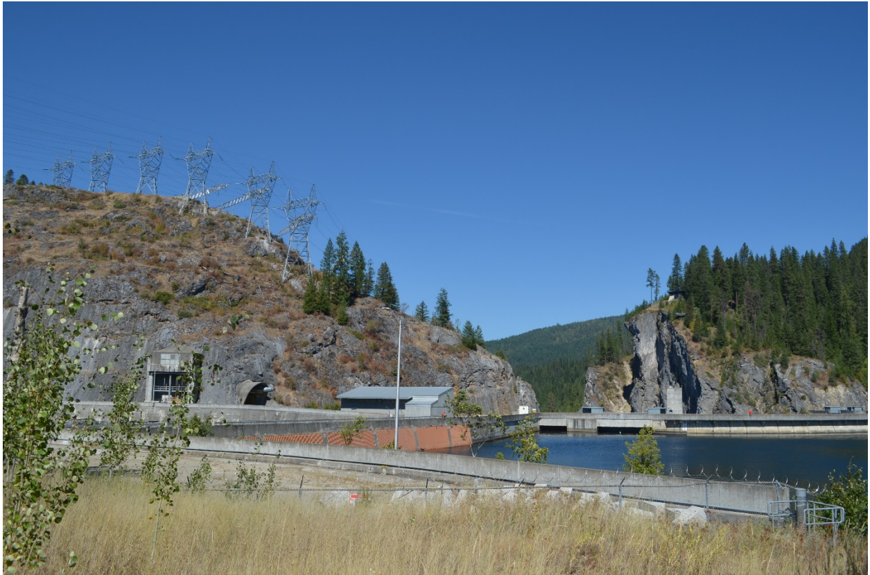
Photo 3 of 25: (WA_PendOreille_BoundaryDam__003) Boundary Dam, Forebay, Towers, camera facing NW, from Forebay Area (A)
