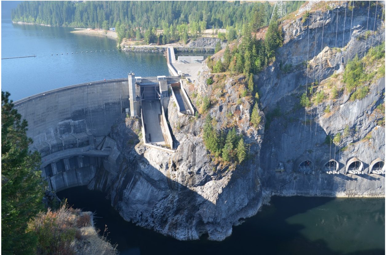
Photo 5 of 25: (WA_PendOreille_BoundaryDam__005) Boundary Dam, Reservoir, Forebay, Transformer Bays (Powerhouse), overview, camera facing SW, from Vista House Overlook (A)
