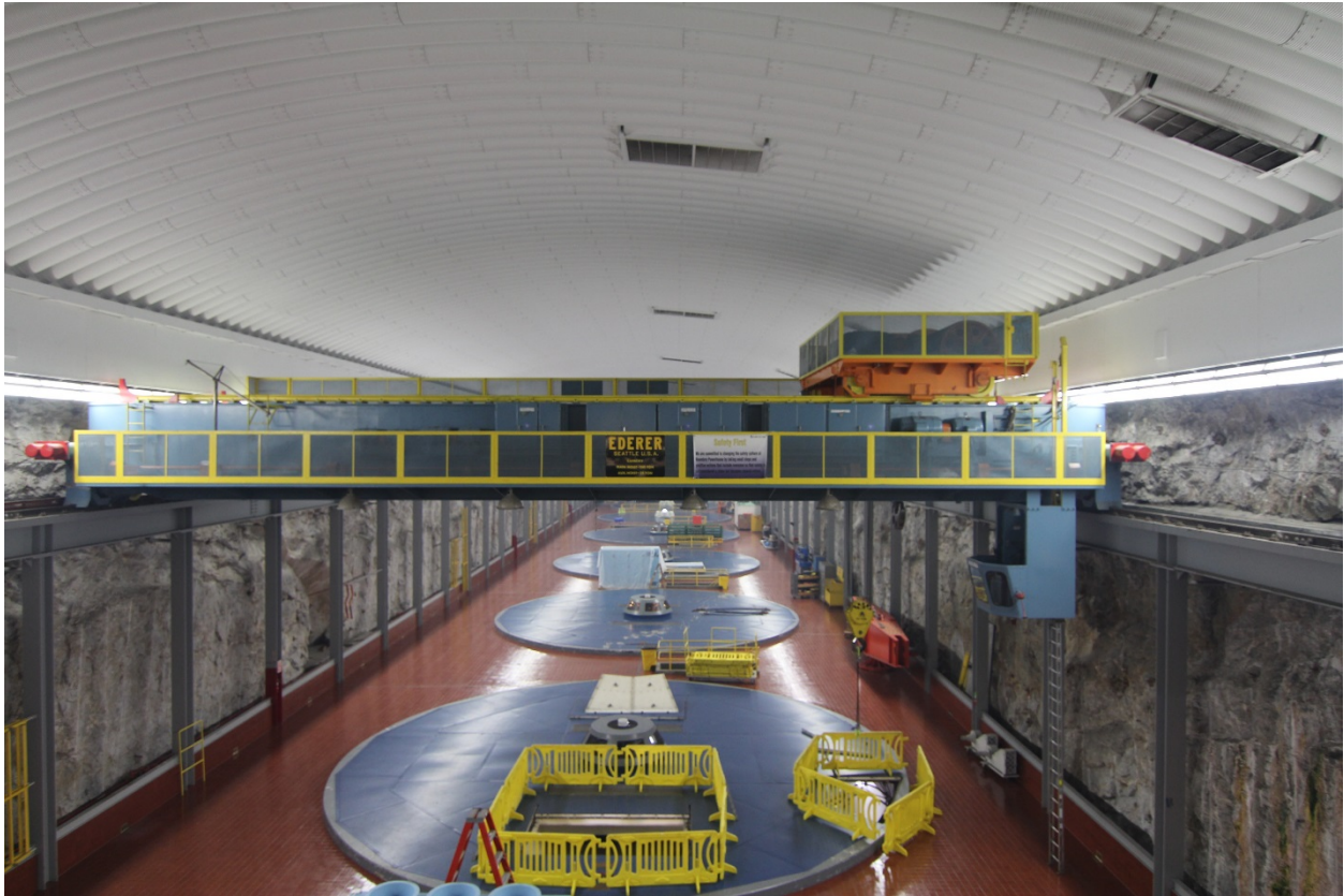
Photo 14 of 25: (WA_PendOreille_BoundaryDam_014) INTERIOR: Boundary Powerhouse/Machine Hall, camera looking E from Visitor Gallery (K)
