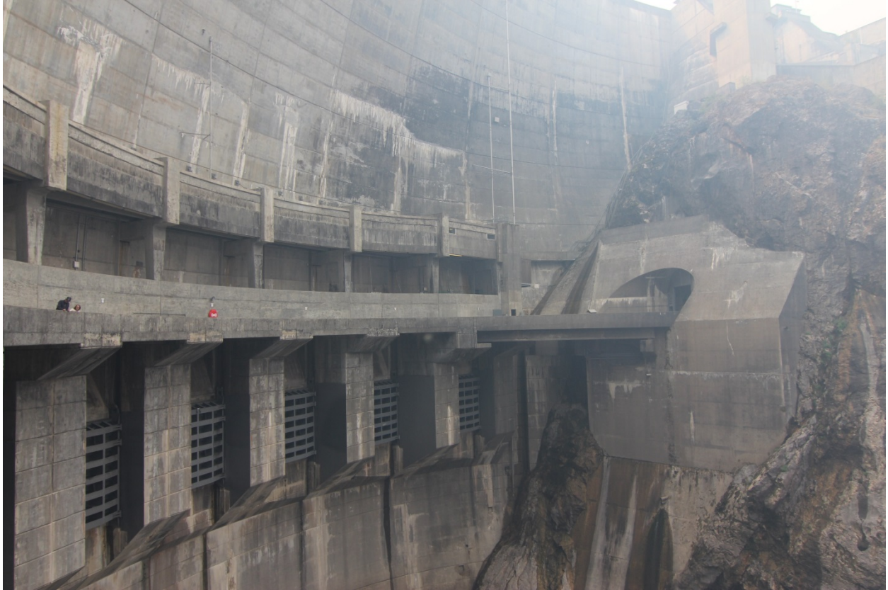
Photo 9 of 25: (WA_PendOreille_BoundaryDam__009) Boundary Dam, downstream face showing sluice gates, cantilever roadway, camera looking SW from Right Abutment at roadway level (K)
