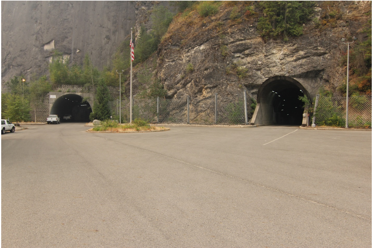
Photo 11 of 25: (WA_PendOreille_BoundaryDam_011) Boundary Dam, Powerhouse Access Tunnels with "Bonnets," camera looking SW from Tailrace Recreation Area/ Access Road (K)
