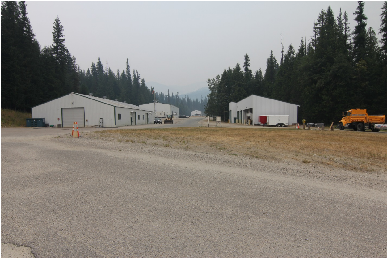
Photo 25 of 25: (WA_PendOreille_BoundaryDam__025) Boundary Dam Operations and Maintenance Service Area, General View, camera looking N from Access Road (K)
