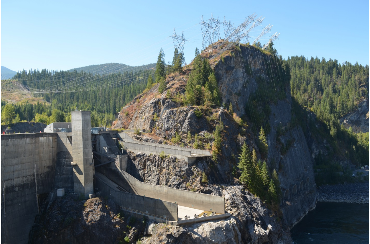
Photo 7 of 25: (WA_PendOreille_BoundaryDam__007) Boundary Dam, Elevator Tower, Left Spillway, Skimmer Gate, Transmission Line, Powerhouse formation, camera-looking West, from Vista House Overlook (A)
