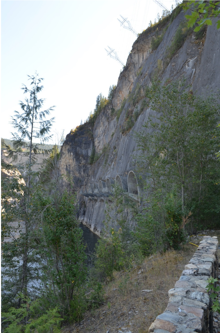
Photo 4 of 25: (WA_PendOreille_BoundaryDam_004) Boundary Powerhouse, Transformer Bays (Bonnets) and Picklefork Towers, camera facing SE from Tailrace (A)
