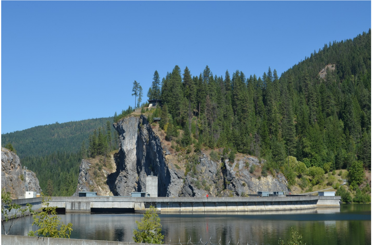
Photo 2 of 25: (WA_PendOreille_BoundaryDam__002) Boundary Dam, Vista House in center, camera facing North, from Forebay area (A)
