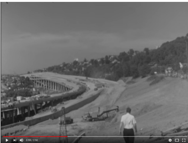
"Construction of Interstate 5 in Seattle, c. 1958" Item 609 , Record Series 9950-01, SMA.
