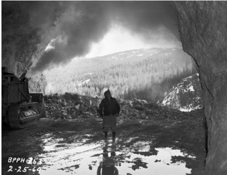
View from Transformer Bay #51 after blast overlooking river, 1964.
