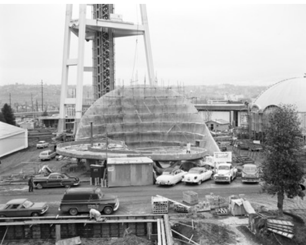
Construction of the Electric Utilities Pavilion for Century 21, February 9, 1962. Item 167574, Seattle Municipal Archives.
