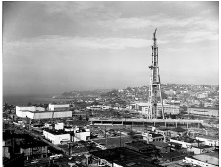
Space Needle Under Construction, 1961
