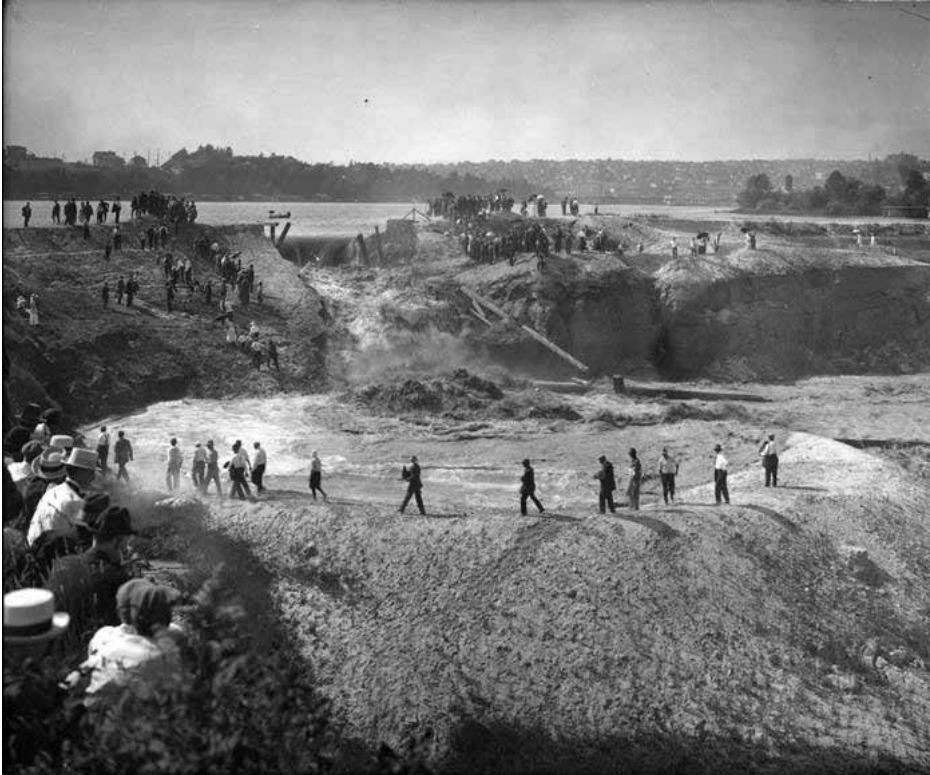
Releasing water from Lake Union into the Montlake Cut, August 26, 1916, Webster & Stevens, 1916. “The Montlake Cut is part of the Lake Washington Ship Canal that connects Puget Sound, Lake Union, and Lake Washington. While digging the Montlake Cut, engineers built a temporary dam to hold back the waters of Lake Union’s Portage Bay .In this photo, a crowd of onlookers watches as the temporary dam at Portage Bay is broken.” Museum of History & Industry Photograph Collection, Image Number : 1983.10.10325
