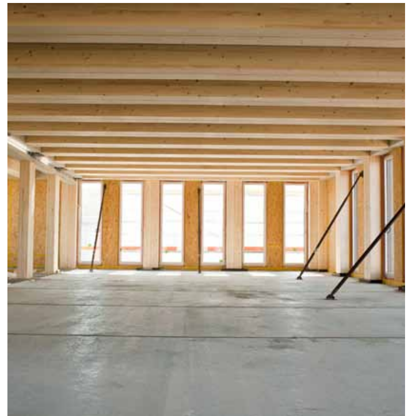
LCT One under construction. Source: CREE Rhomberg
