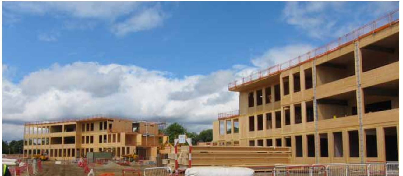
The City Academy under construction
