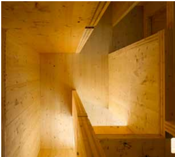
Stadthaus under construction. Source: Waugh Thistleton/KLH UK
