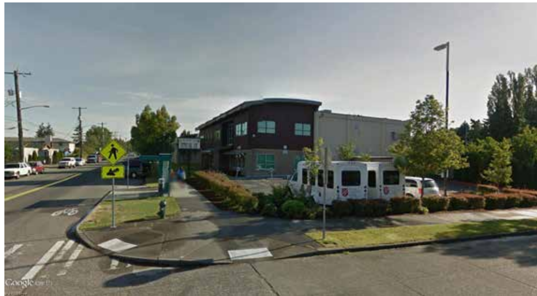
A Salvation Army building @ corner of SW Barton and 16th Ave SW, recently renovated in 2004 to include a community center, gymnasium, and chapel.
