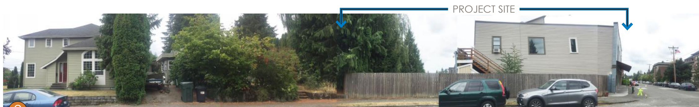
2 Looking into the site from NE 68th St
