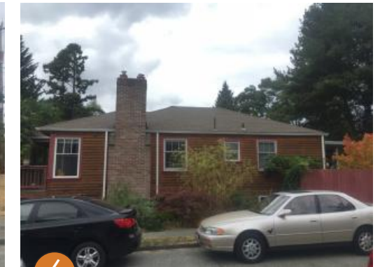
6 Single family north of the site
