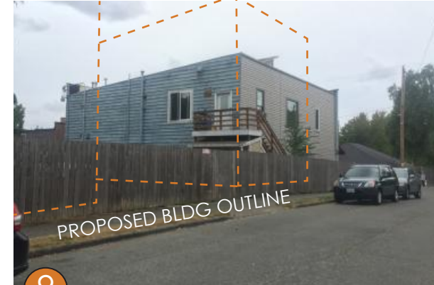
9 Looking into the site from NE 68th St
