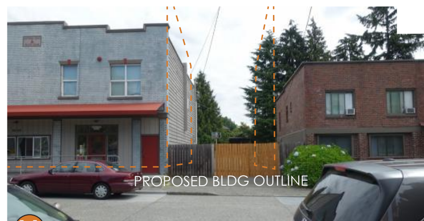
11 Looking into the site from Ravenna Ave NE
