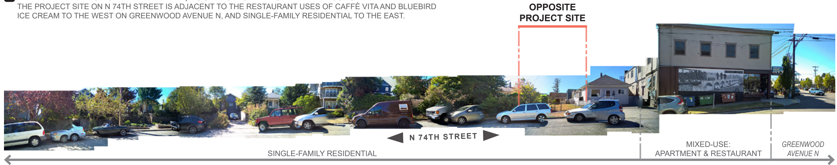
B STREET VIEW ALONG N 74TH STREET, LOOKING SOUTH OPPOSITE PROJECT SITE OPPOSITE THE PROJECT SITE ON N 74TH STREET CONSISTS MOSTLY OF SINGLE-FAMILY RESIDENTIAL, WITH JUST ONE MIXED-USE BUILDING CONTAINING APARTMENTS ON TOP OF HERKIMER COFFEE ANCHORING THE CORNER AT GREENWOOD AVENUE N.
