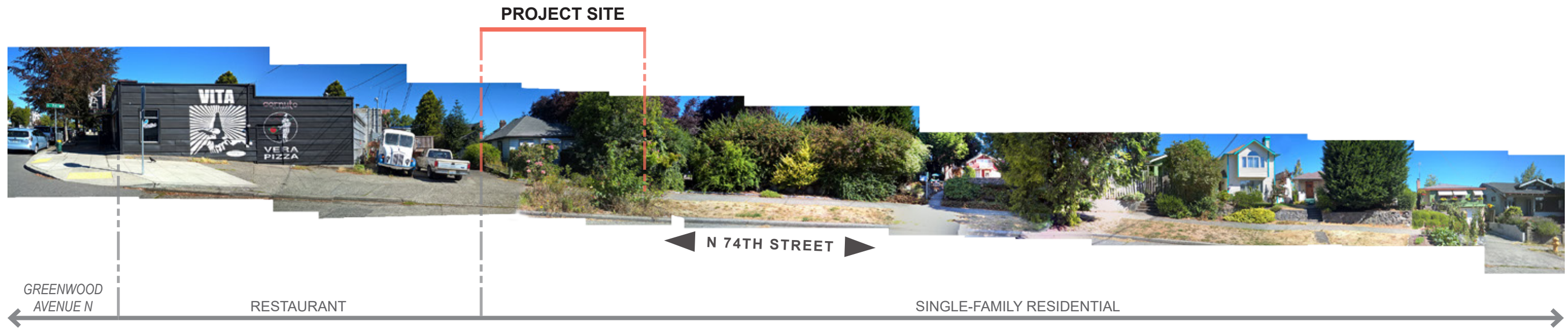
A STREET VIEW ALONG N 74TH STREET, LOOKING NORTH TOWARDS PROJECT SITE THE PROJECT SITE ON N 74TH STREET IS ADJACENT TO THE RESTAURANT USES OF CAFFÈ VITA AND BLUEBIRD ICE CREAM TO THE WEST ON GREENWOOD AVENUE N, AND SINGLE-FAMILY RESIDENTIAL TO THE EAST.
